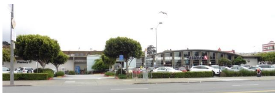
Figure 28: Front of Safeway, facing south.
