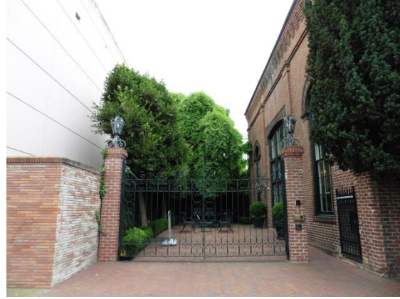
Figure 21: Large iron gate and Landmark No. 58 (right) with driveway in foreground and side patio in background, facing south.
