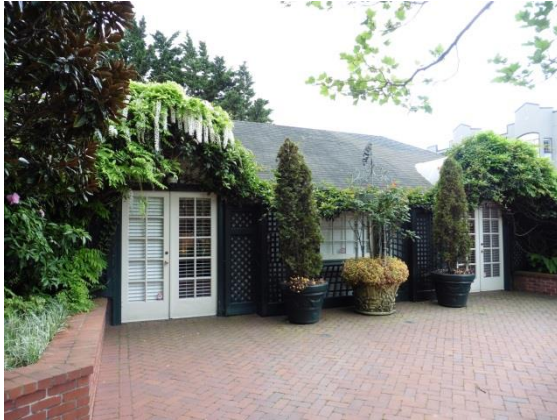
Figure 10: Rear façade, facing southwest.
