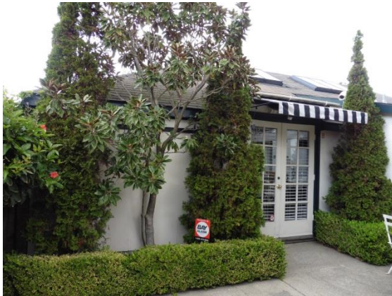
Figure 4: Western-most bay, facing north.
