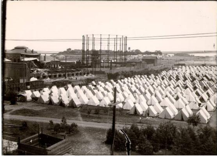
Figure 38: 1906 photograph of Lobos Square Refugee Camp, showing the damaged North Beach Station in the background.
