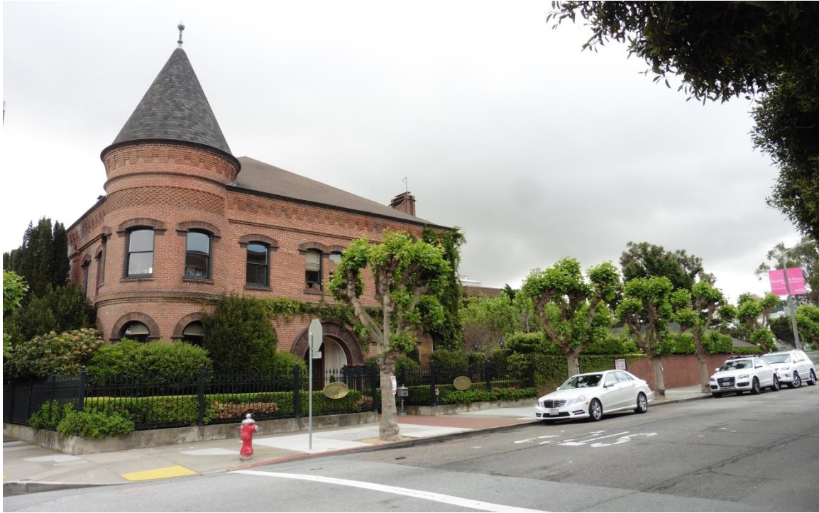
Figure 13: Landmark No. 58 (left) and subject building (right), facing southeast.
