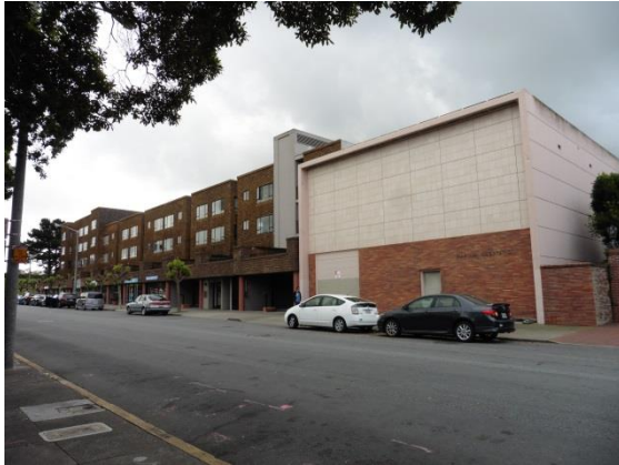
Figure 24: Marina Substation and the apartment complex, facing southwest.
