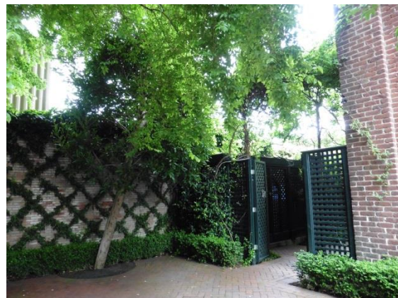
Figure 19: Lattice door and south brick wall of side patio, facing southwest.
