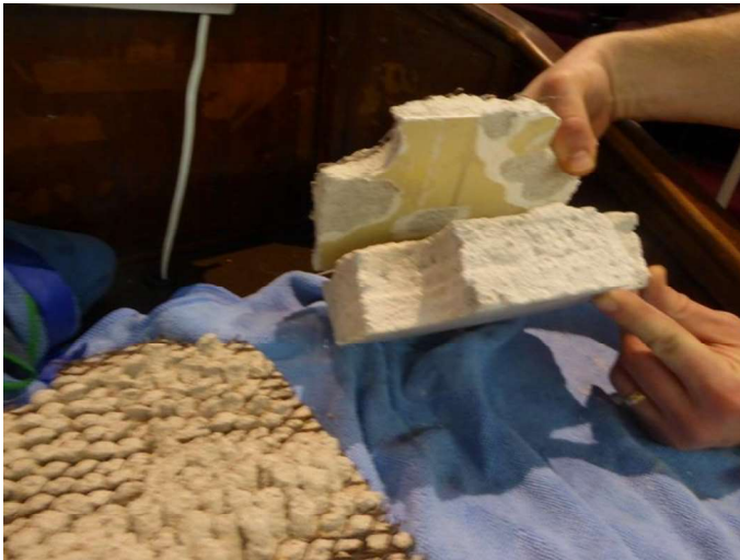
Figure 5: Access panel from pilaster shows finish paint between layers of plaster.
