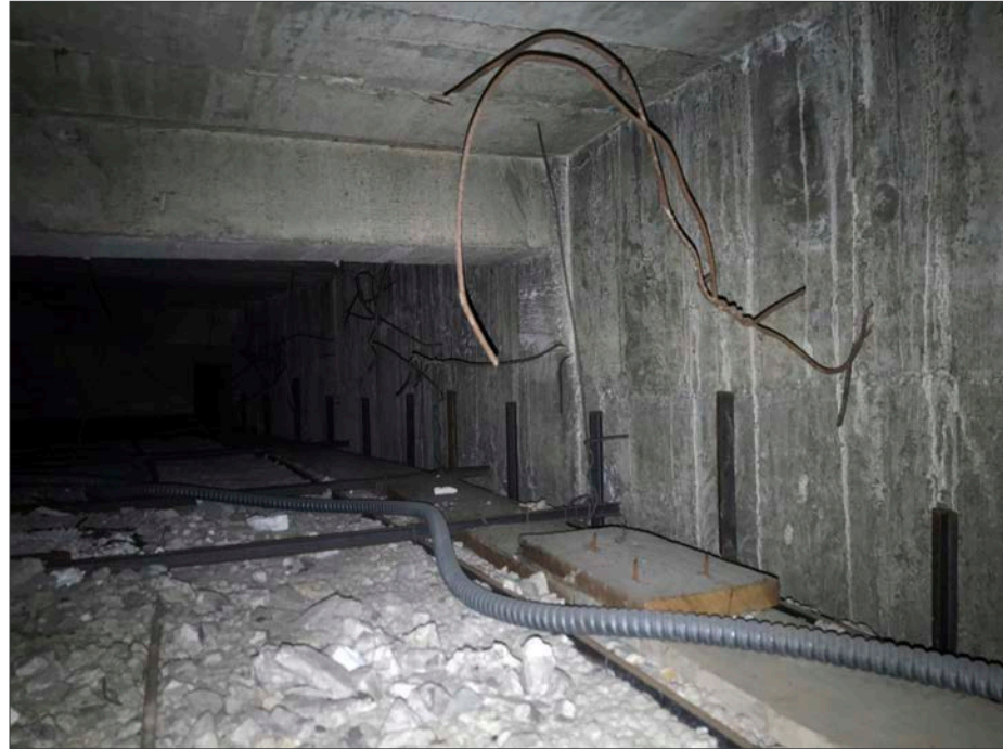
Ceiling above Fresco 3. Note the ceiling framing and the vertical furring channels of the fresco supports. Photo by Tuan and Robinson.
