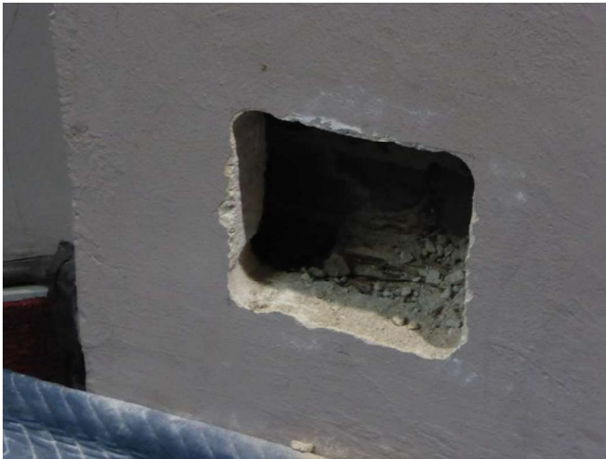
Figure 4: Decorate plaster pilaster
