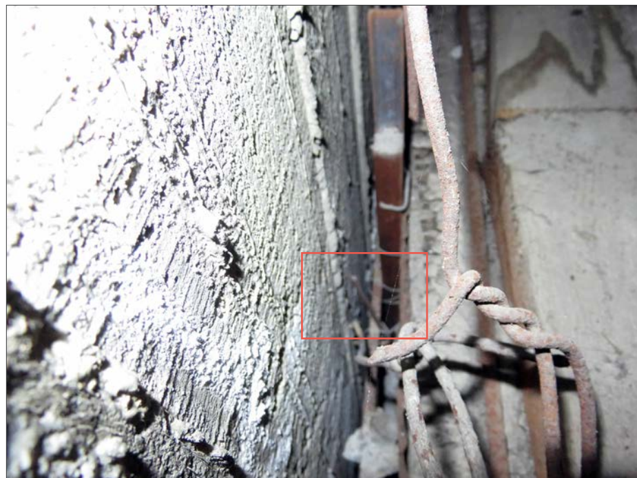
View behind Fresco 3 from above. Note the form tie used to attach the vertical support to the wall.
