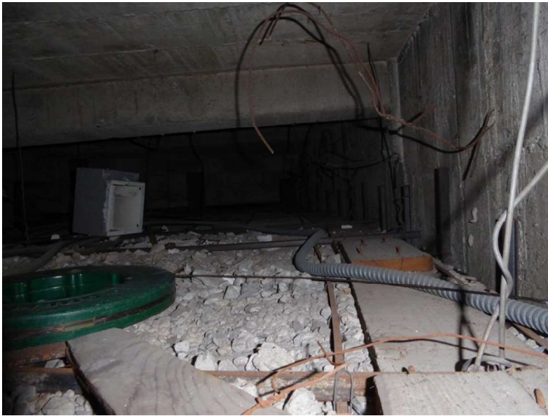
Figure 2: Image looking across plenum space above fresco wall, showing concrete rear wall, ceiling and lathe and plaster soffit.
