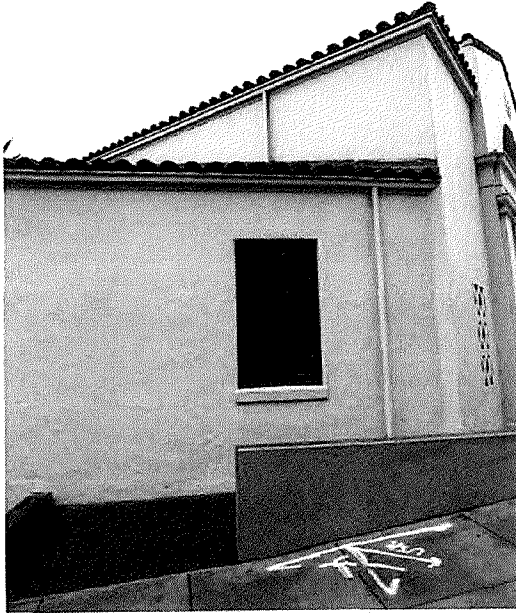
Figure 12 - The downspout from the upper roof sheds water onto this area of the lower roof, which bypasses the gutter and spills onto the ADA ramp into the Entry Pavilion. Photo by Page & Turnbull, 2017.
