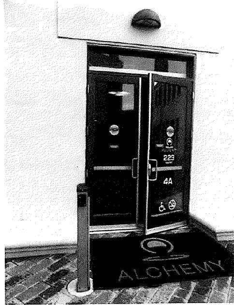
Figure 13 - The ADA pushplates at these courtyard doors only open the door this much. Photo by Page & Turnbull, 2017.
