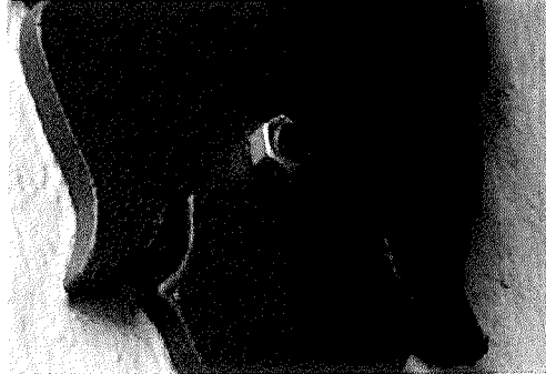
Figure 15 - (above) A rusted bolt anchoring the sconces. Photo by Page & Turnbull, 2017
