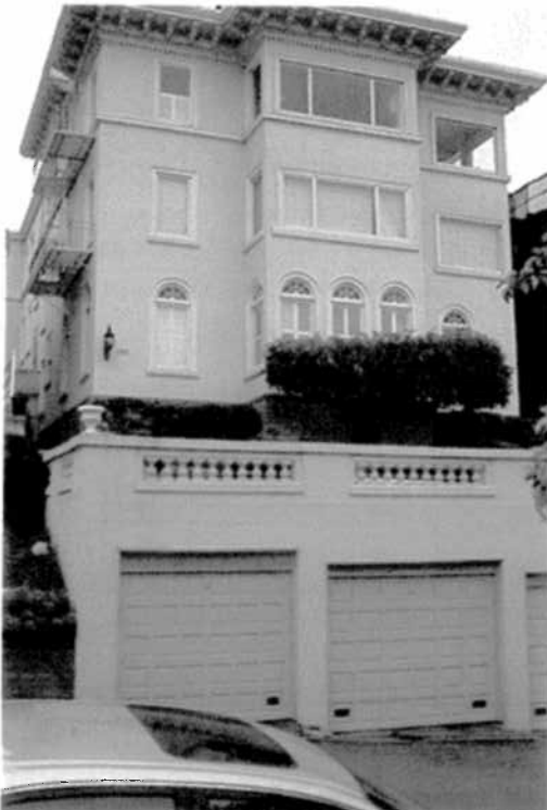
LOOKING WEST FROM 24 TH AVE. TOWARDS THE GARAGES OF 155 – 24 TH
