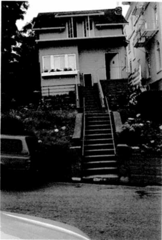
LOOKING WEST FROM 24 TH AVENUE TOWARDS 157 – 24 TH
