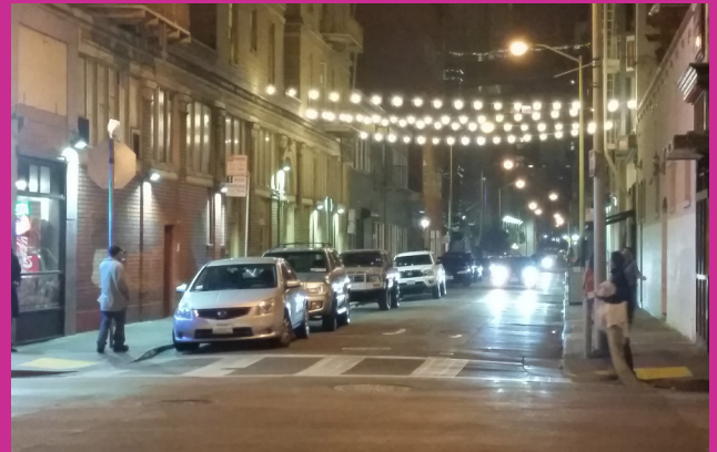
Stevenson Street Lighting Project
