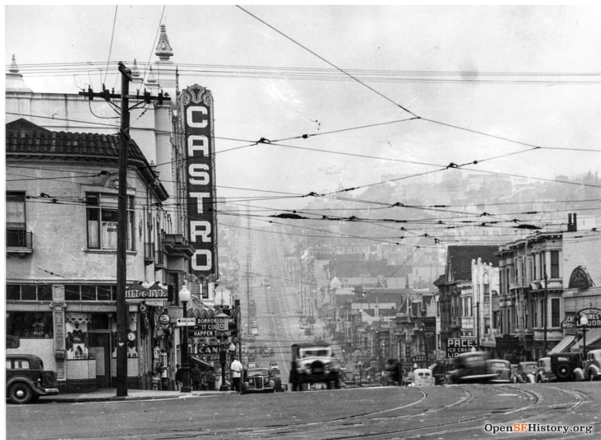
1939 photo of Castro Street looking south from Market Street. Image Source: Image Source: OpenSFHistory / wnp4.1284
