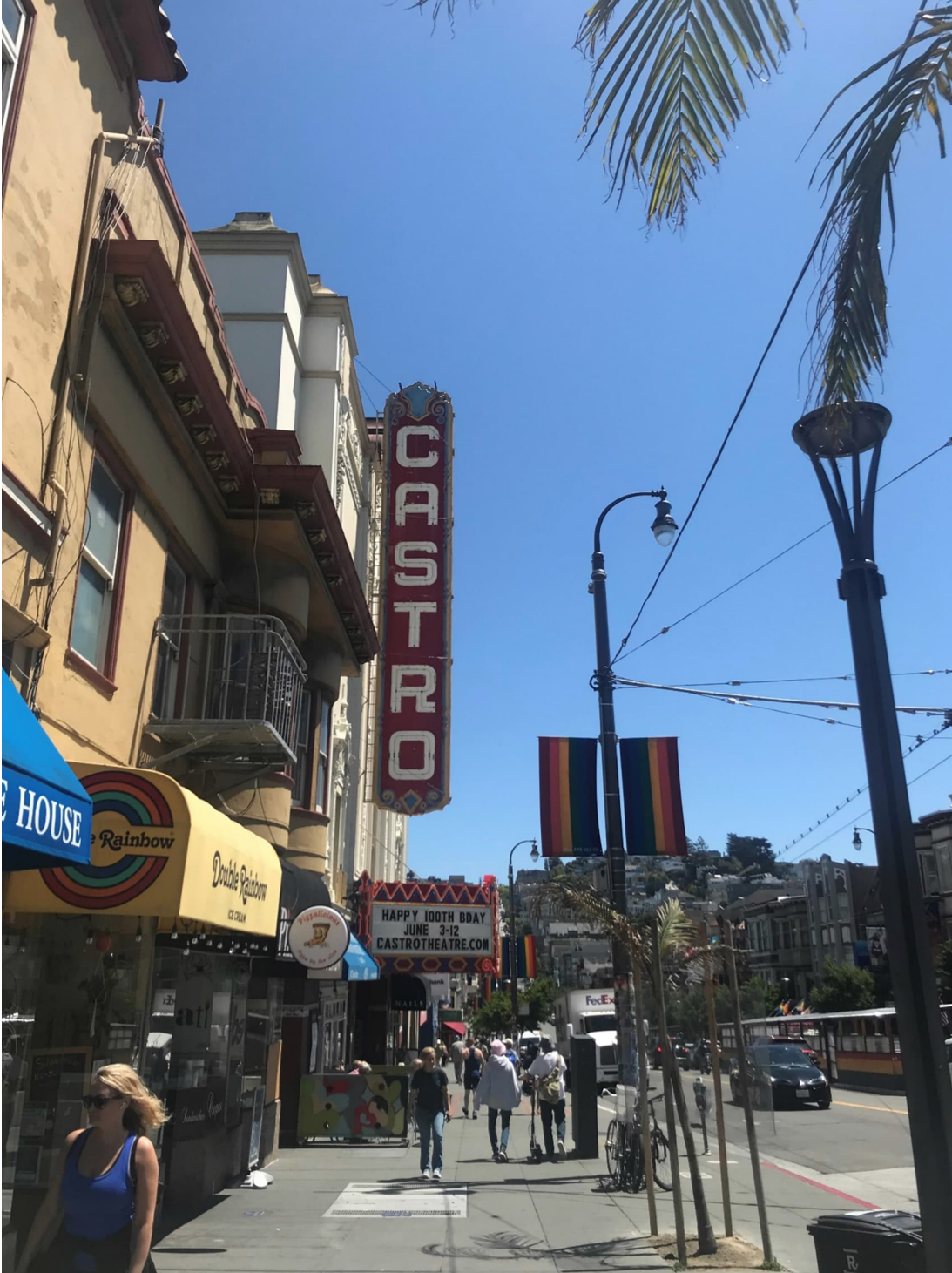
Vertical blade sign and marquee, northern elevation Image Source: SF Planning Department, 2022
