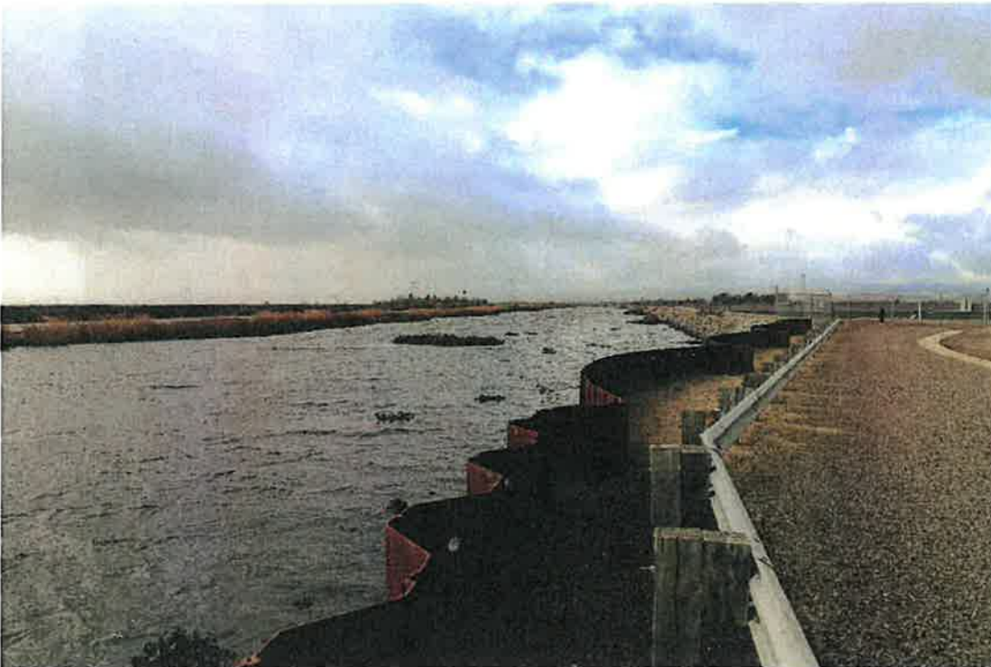
Victoria Canal/Middle River point of diversion/fish screen on 1/22/21, looking west
