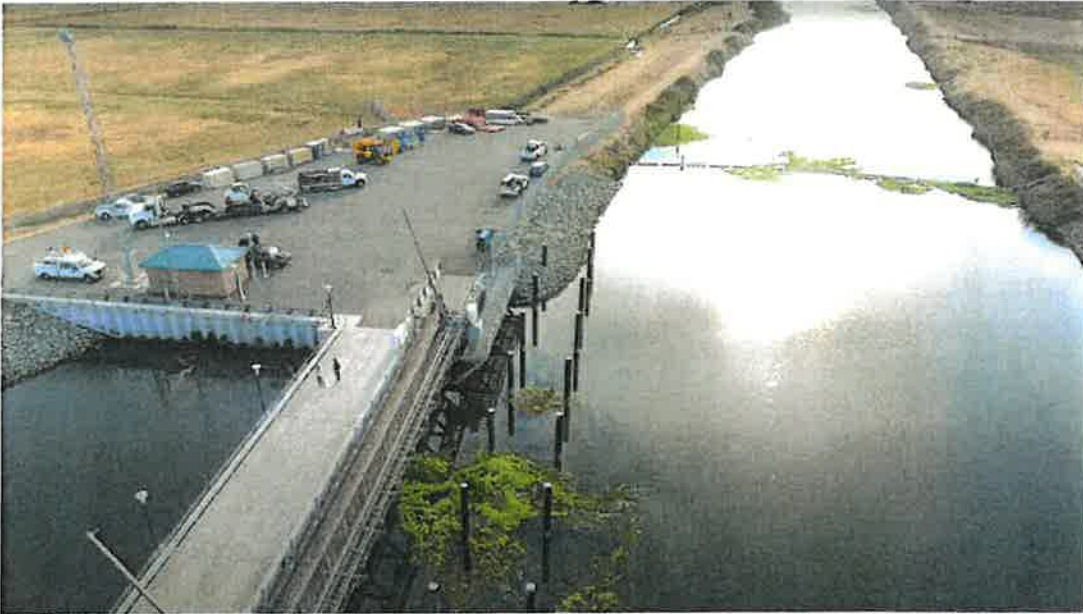
Rock Slough point of diversion/fish screen on 12/30/2020, looking east
