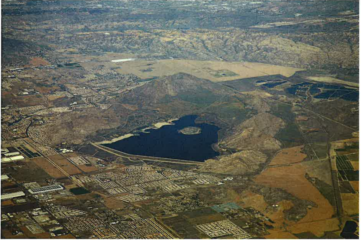
Perris Lake and Dam and adjacent lands within State Water Project service area – point of rediversion, June 2013, looking northeast
