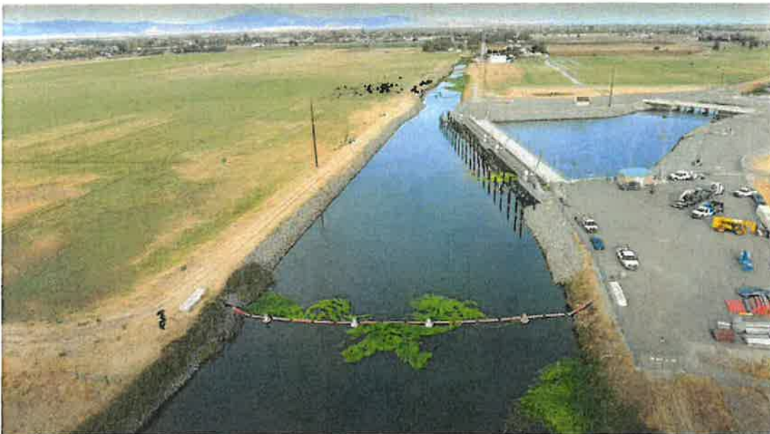
Rock Slough point of diversion/fish screen on 12/30/2020, looking west
