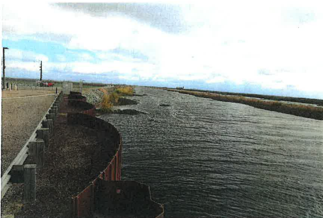
Victoria Canal/Middle River point of diversion/fish screen on 1/22/21, looking east
