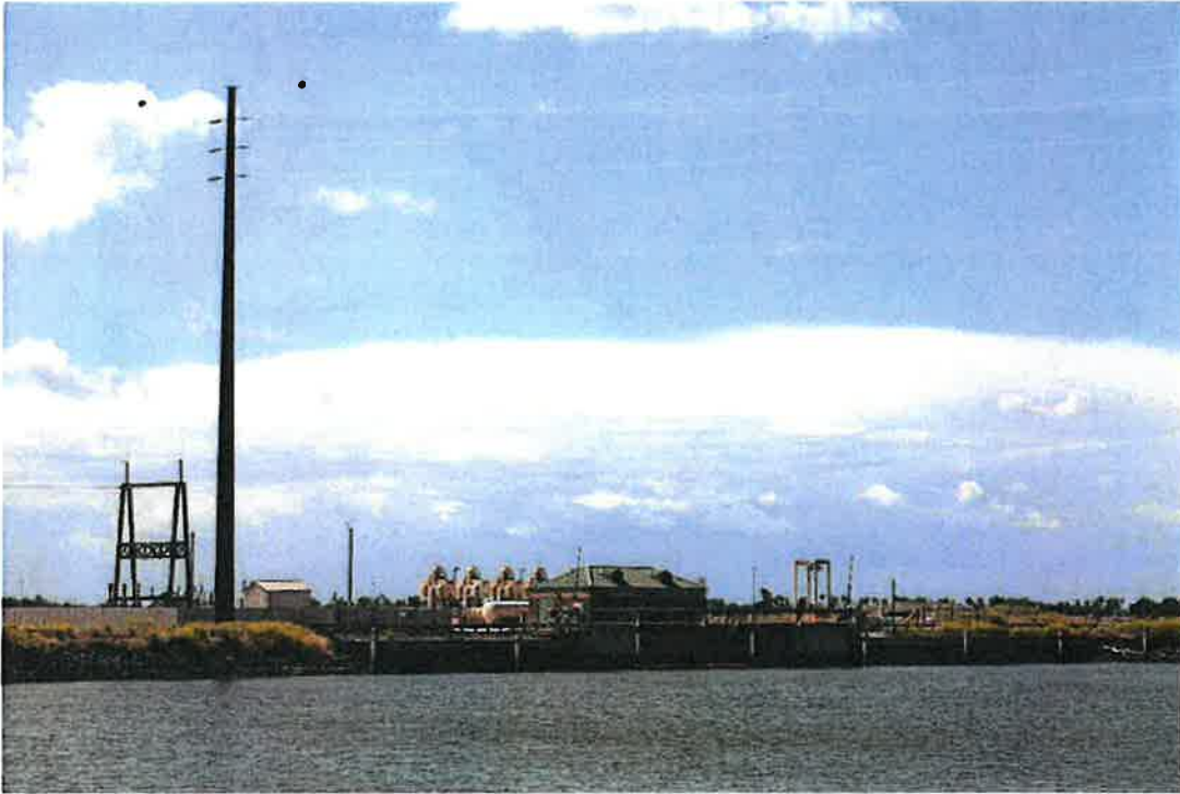
Old River point of diversion/fish screen on 5/14/17, looking northwest
