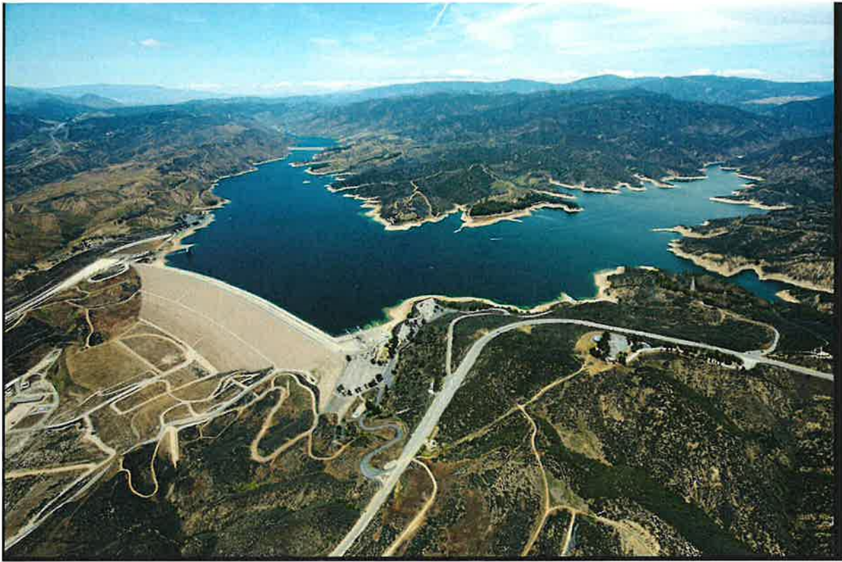
Castaic Lake and Dam – point of diversion, May 2014, looking northwest
