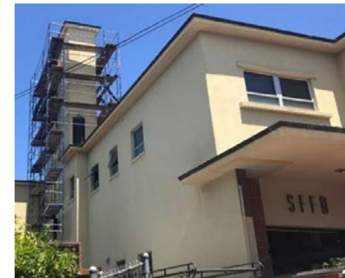
Fire Station - Seismic Hose Tower
