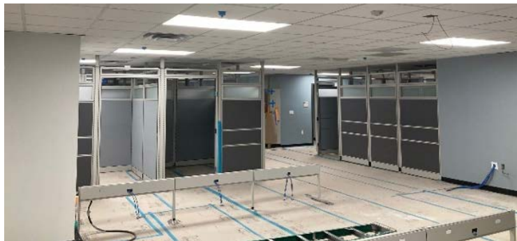
ZSFG 6H Surge – New workstations installation
