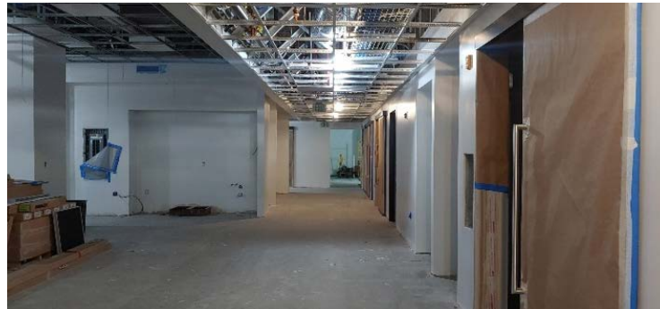
ZSFG Rehab – New Exam Rooms
