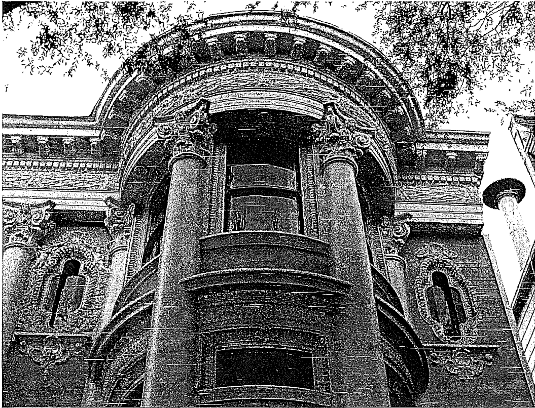
Figure 18: Bay flanked by oval windows in elongated quatrefoil surrounds (south window has a simpler surround).
