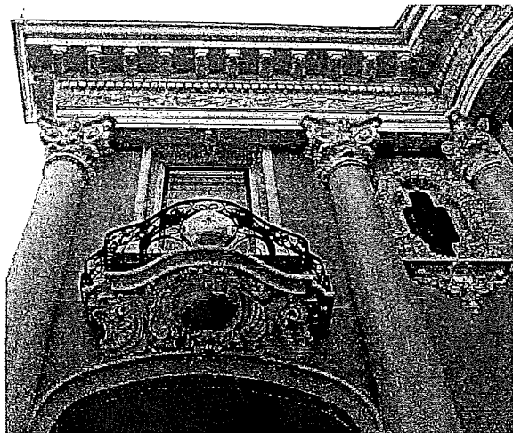
Figure 16: North side of primary façade.
