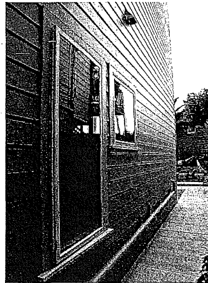
Figure 23: First story fenestration of south façade, facing east.
