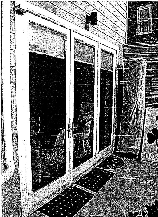
Figure 31: North side ground level.
