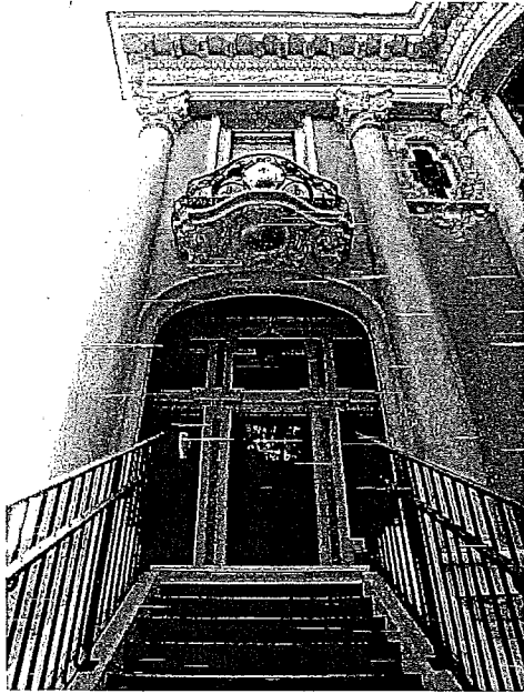
Figure 14: Molded balcony with flanking engaged columns.
