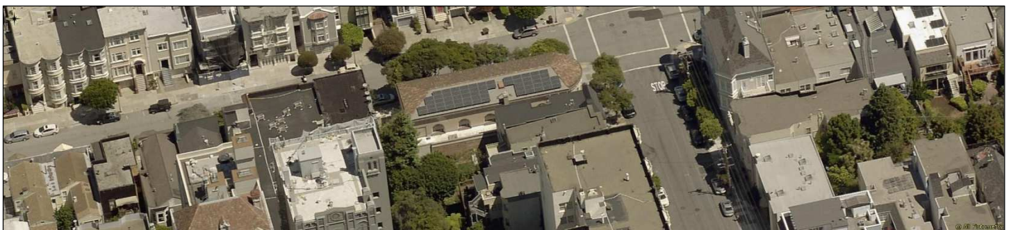
FIGURE 5: AERIAL VIEW OF THE CURRENT CONDITIONS AS OF 07/06/2020.
