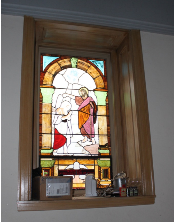
FIGURE 16 (LEFT). CHURCH: BAPTISTRY, INTERIOR WINDOW TRIM, 2016.
