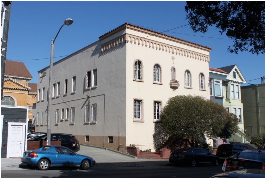
FIGURE 47. CONVENT LOOKING NORTHEAST FROM OAK ST., 2015.
