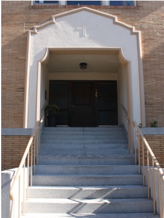
FIGURE 39 (LEFT). RECTORY: MAIN ENTRANCE, 2015.
