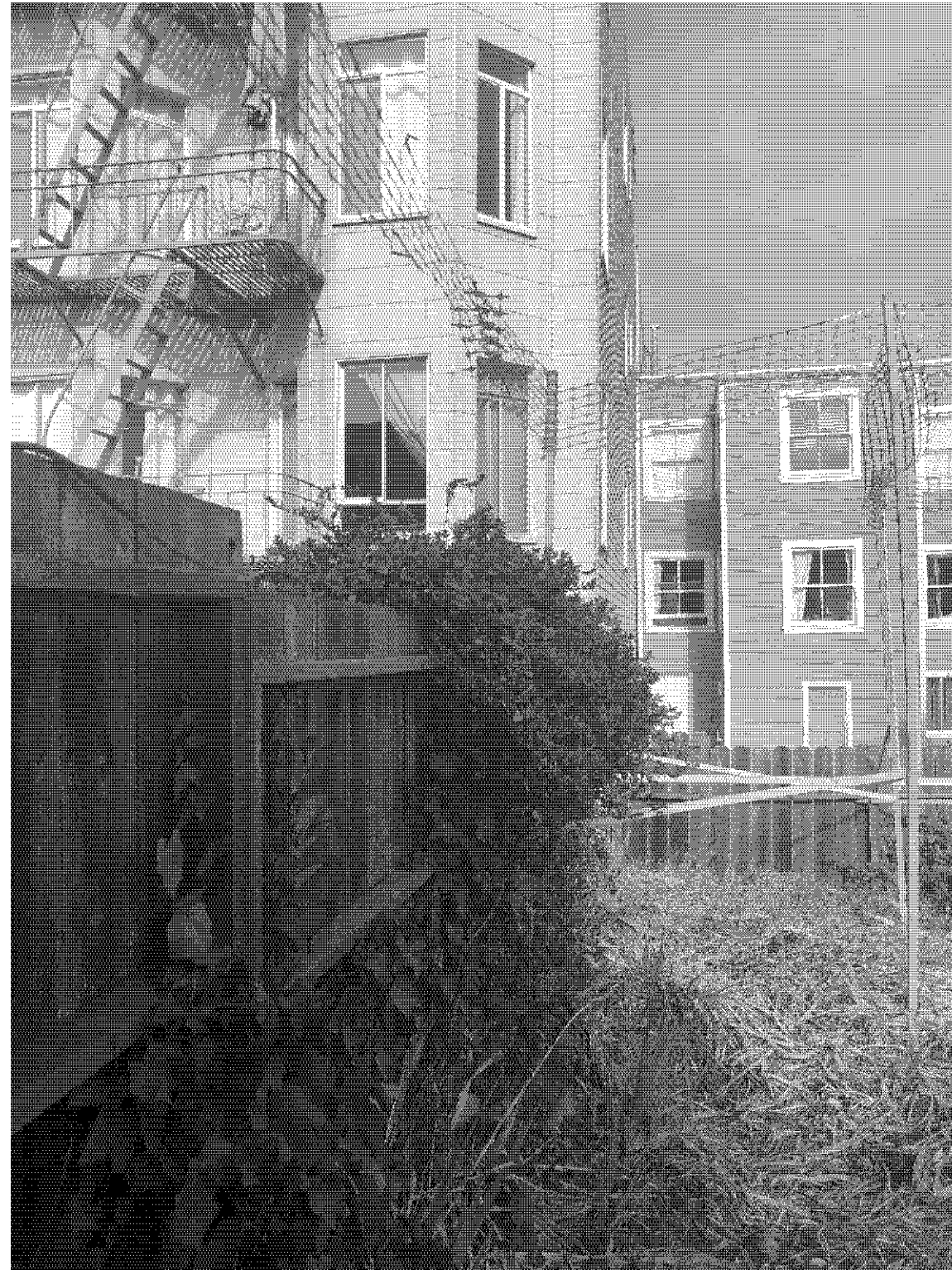
Exhibit L: Unit 3, prior to additional setback at 2nd floor. First floor at fence height
