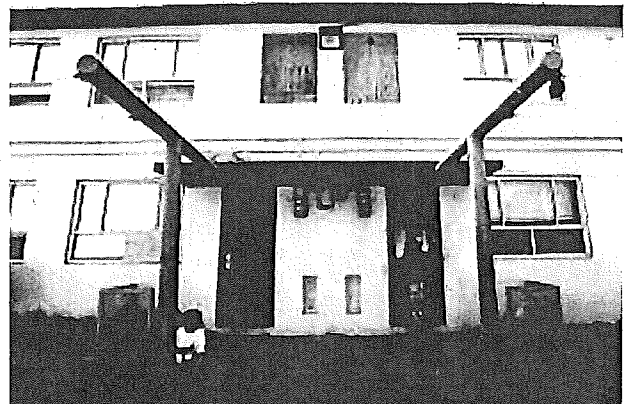
Hunters View public housing before HOPE SF transformation
