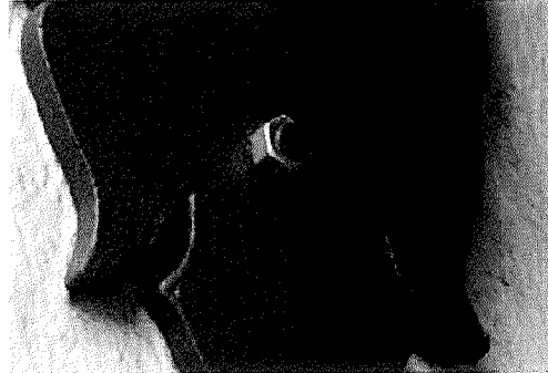
Figure 15 - (above) A rusting bolt anchoring the sconces. Photo by Page & Turnbull, 2017
