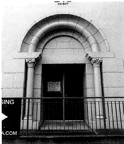
Figure 21 - The street entry with replaced doors. Photo by Page & Turnbull, 2017
