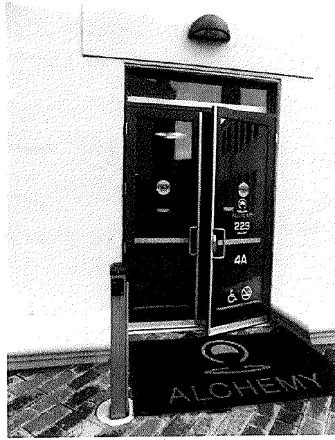
Figure 13 - The ADA pushplates at these courtyard doors only open the door this much. Photo by Page & Turnbull, 2017.
