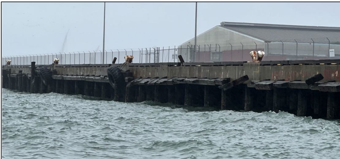
Figure 5. Fendering and Mooring Points at Pier 80 – Existing Condition
