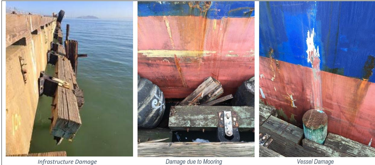
Figure 1: Typical Damage at Pier 80
