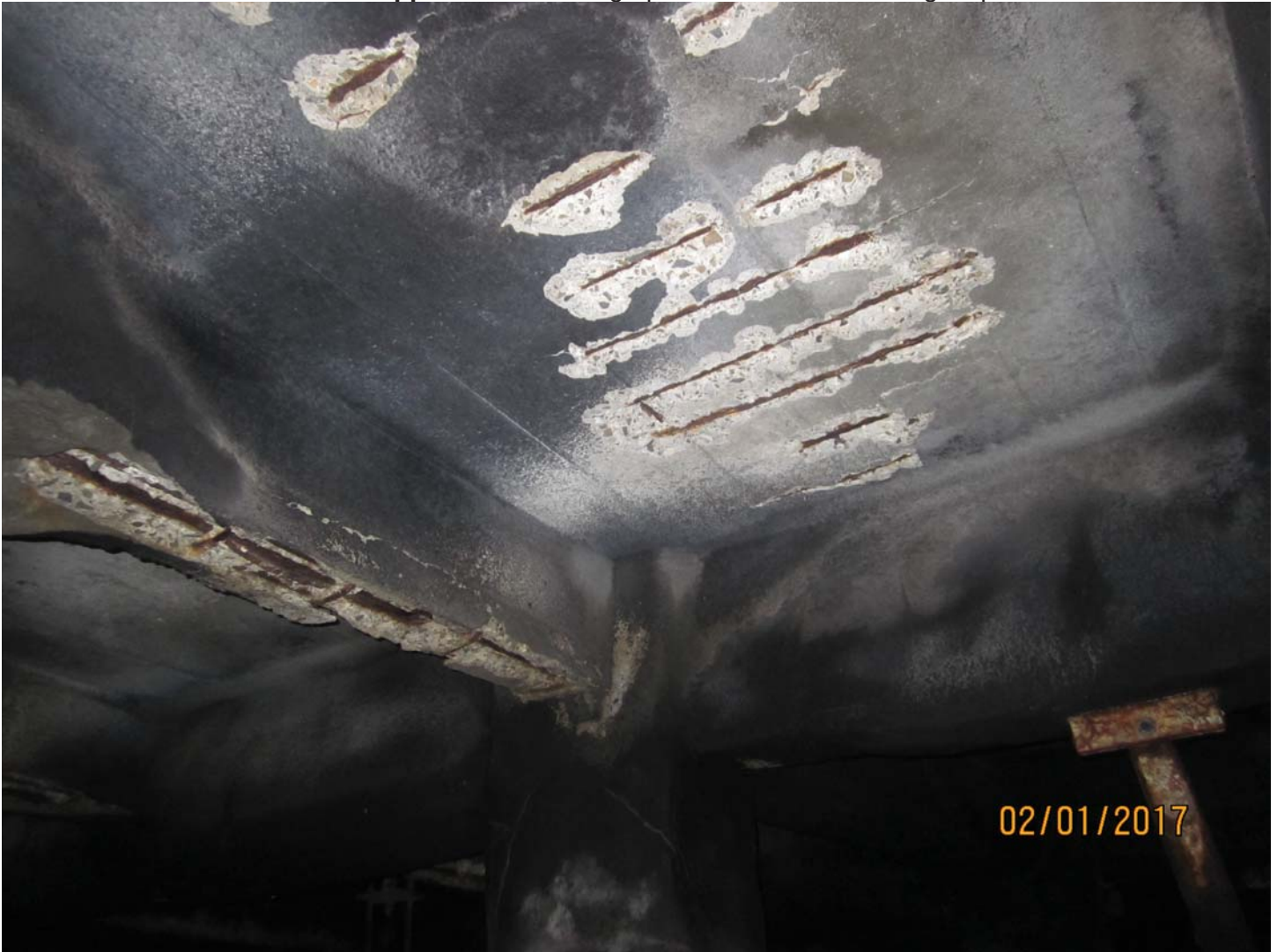
Photo 5. Deck under north end of bulkhead building has more spalls in shotcrete repair due to rebar corrosion
