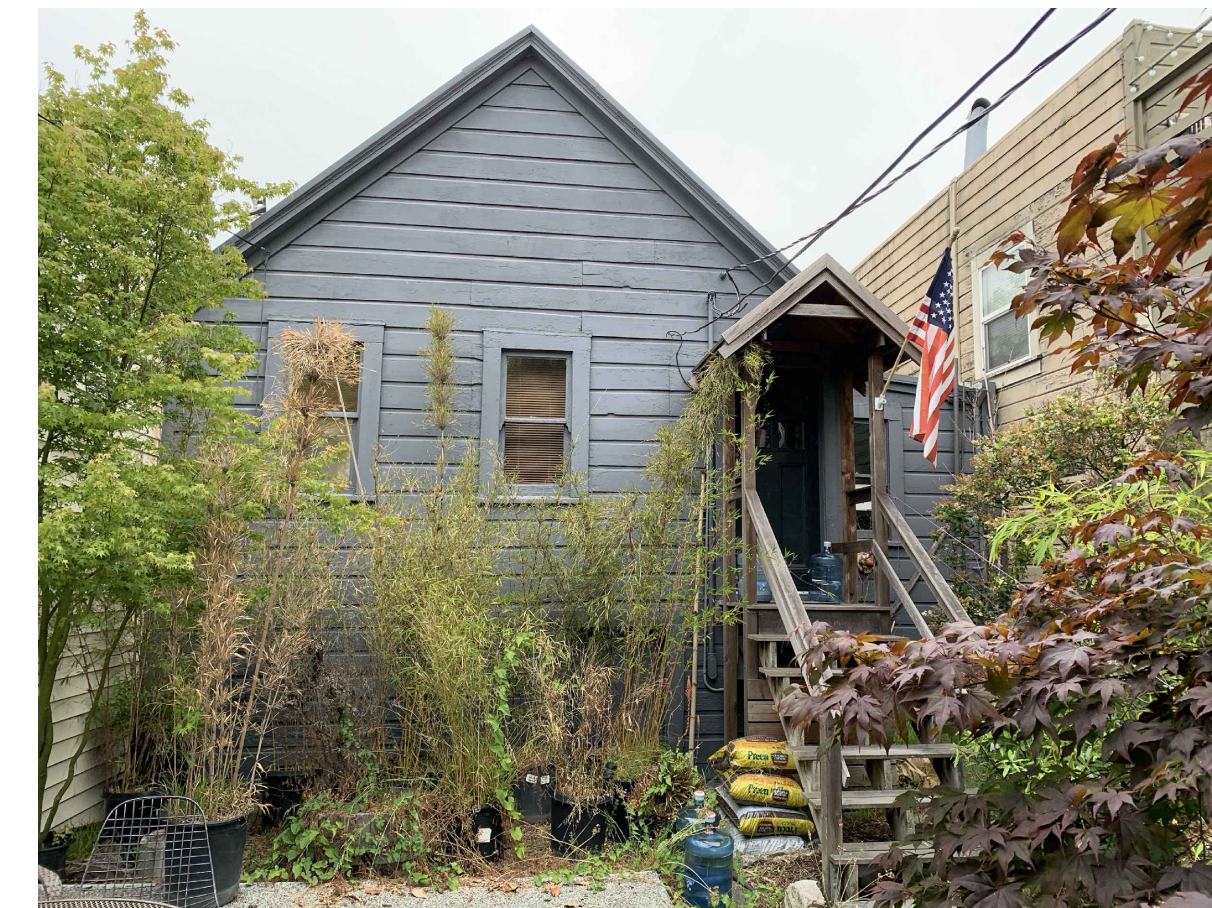
FRONT VIEW: FROM FRONT YARD
