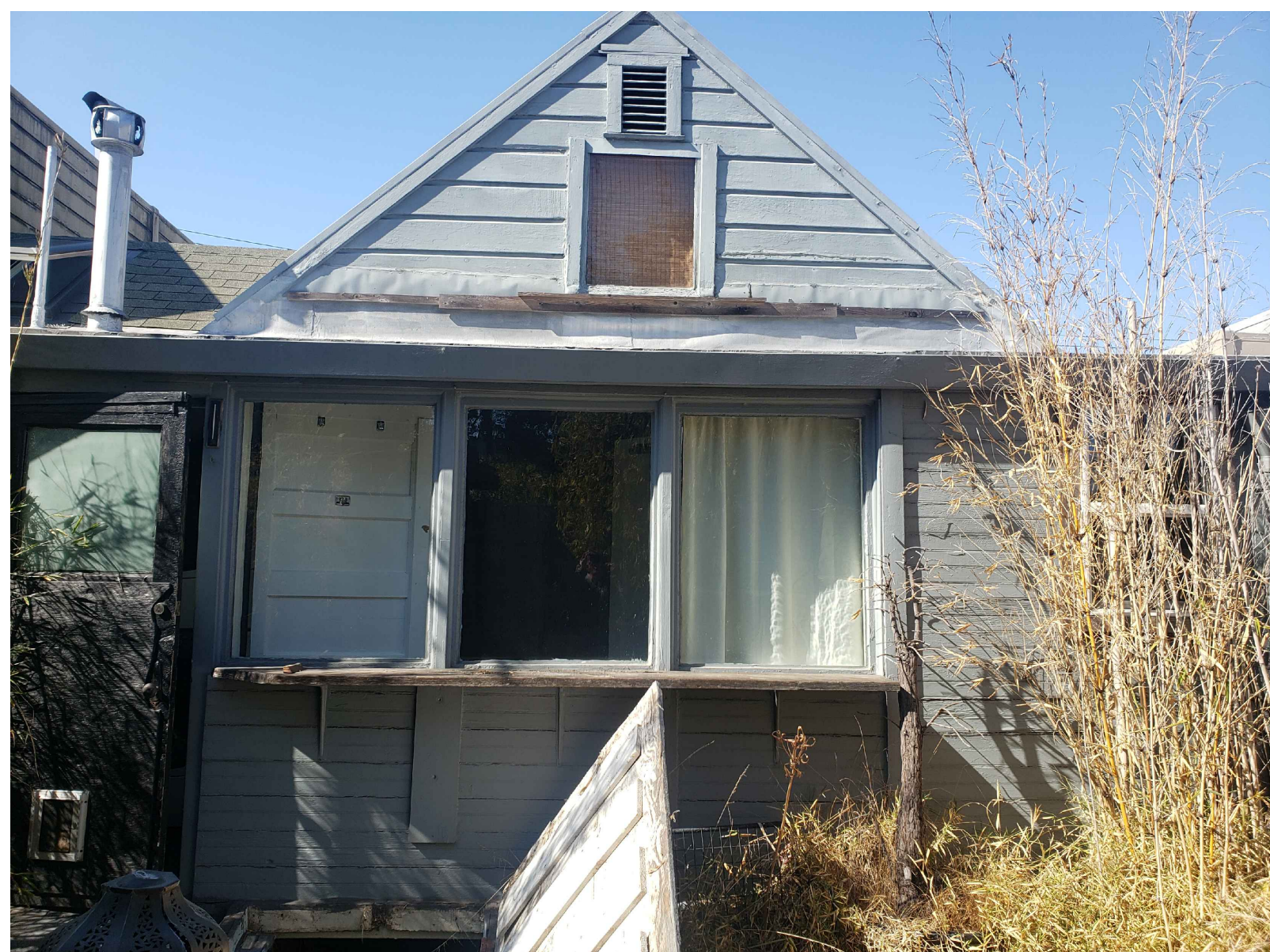
PHOTO 'E' - VIEW OF REAR FACADE
