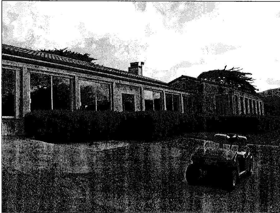
Photograph 10: West side of clubhouse, camera facing southeast 3/4/2010
