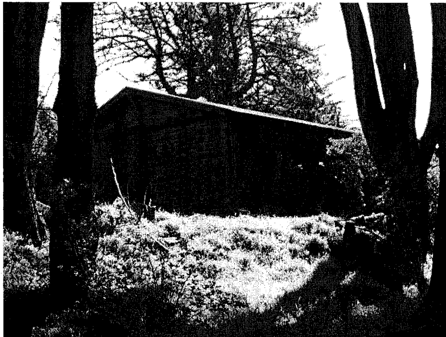
Photograph 11: Maintenance building, camera facing southeast, 3/4/2010
