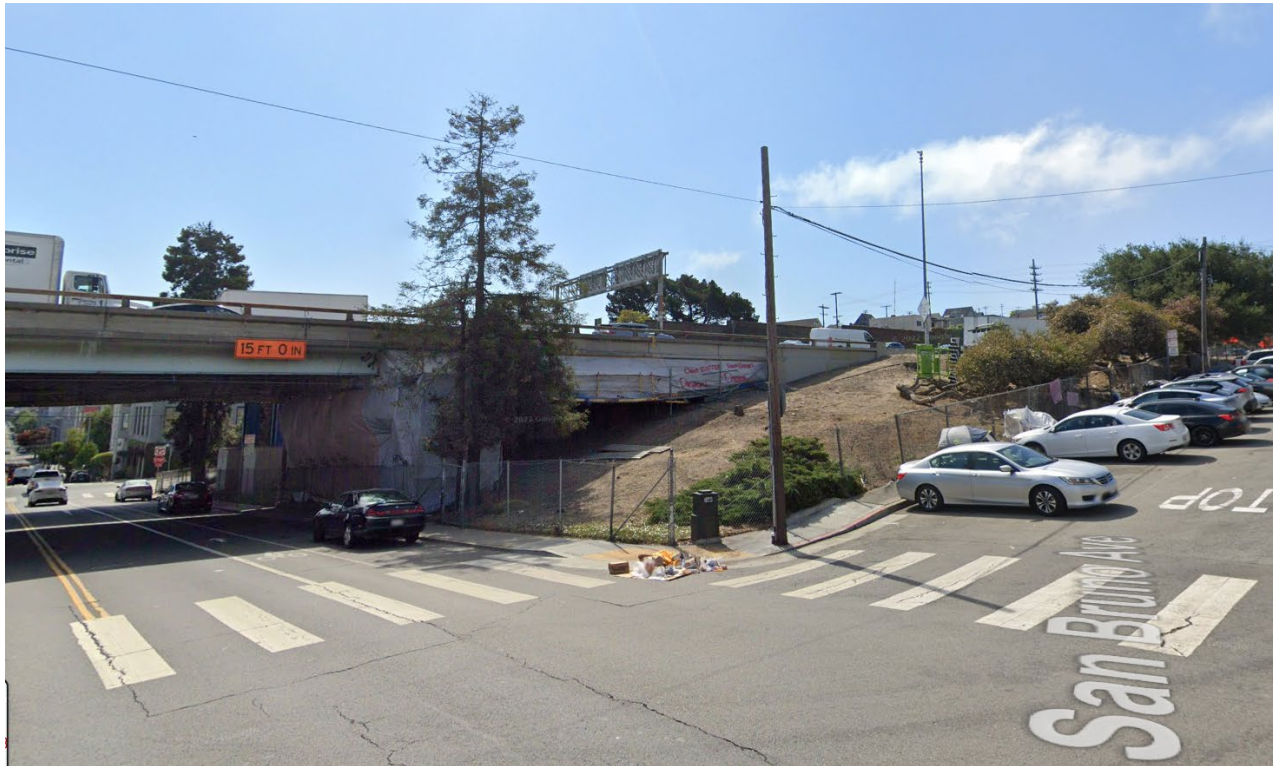
Corner of 17 th Street and San Bruno Avenue facing the Potrero Gateway Park
