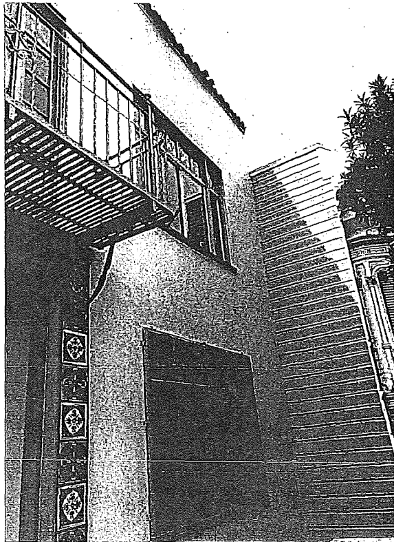
Detail at front façade, view southwest.
