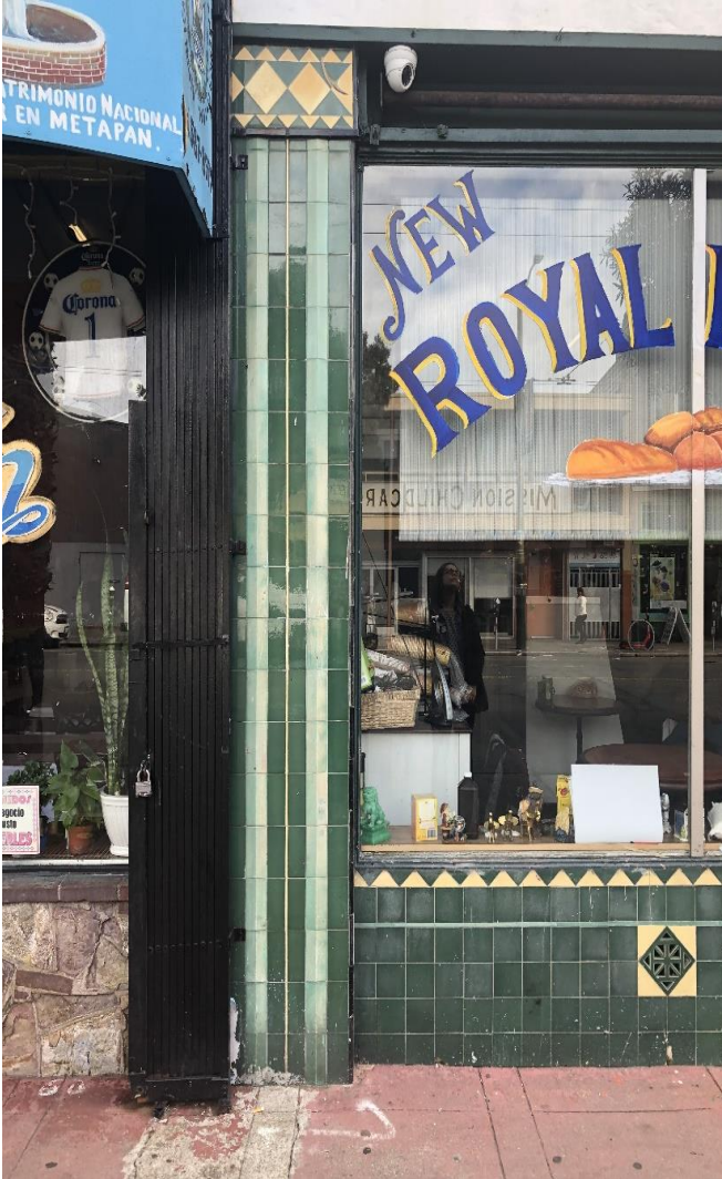
Original ceramic tile pier, bulkhead, and storefront glazing at 4773 Mission Street, January 2020.
