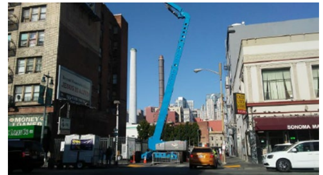
Construction of a traffic signal on Jessie and 6 th Streets.
