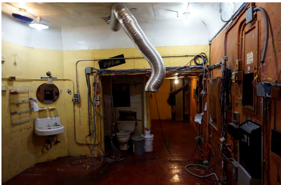
Clay Theatre, Second Floor, Projection Room, 2020. Source: DNM Architecture
