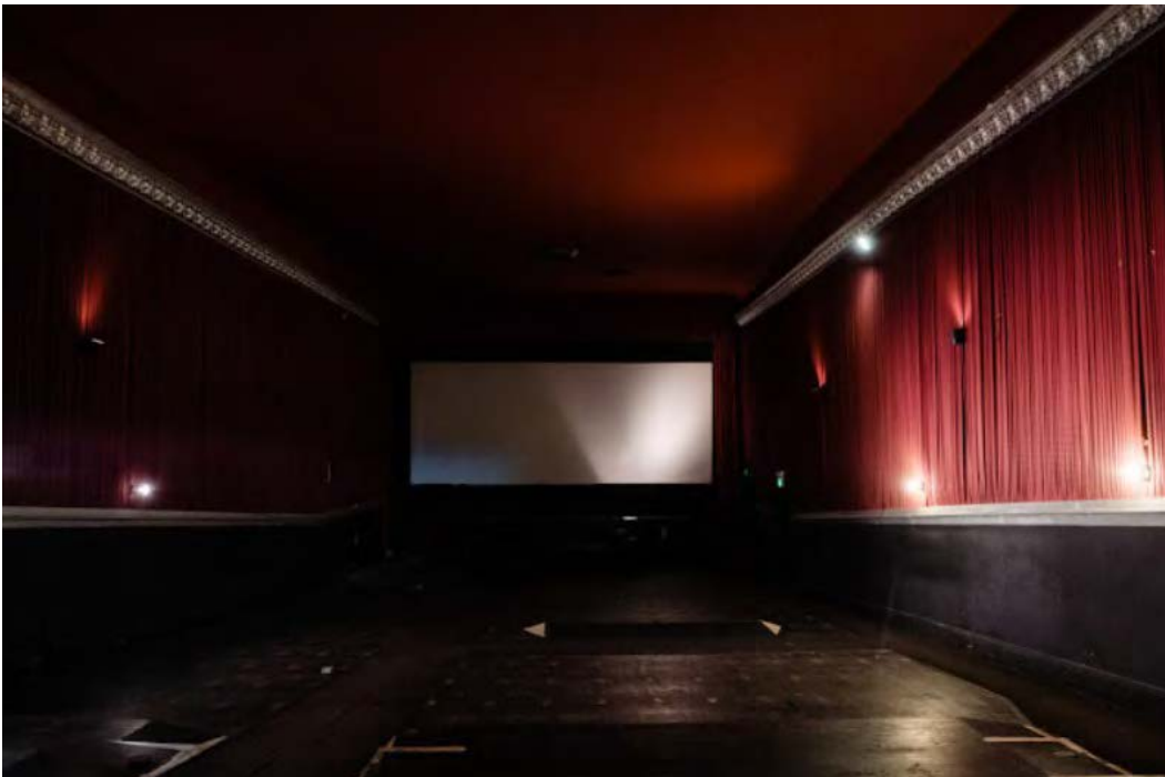
Clay Theatre, Auditorium, seats removed, 2020. Photo by Nick Otto in Sam Whiting, "SF supervisor hopes a law will save historic Clay Theatre, other single screens," San Francisco Chronicle , March 9, 2020.
