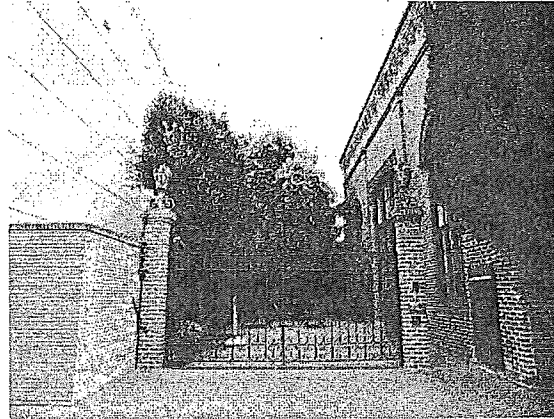
Figure 21: Large iron gate and Landmark No. 58 (right) with driveway in foreground and side patio in background, facing south.
