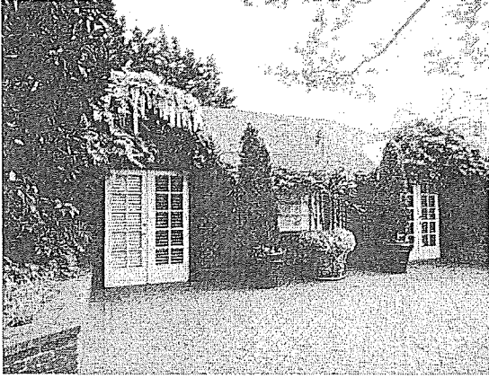
Figure 10: Rear façade, facing southwest.
