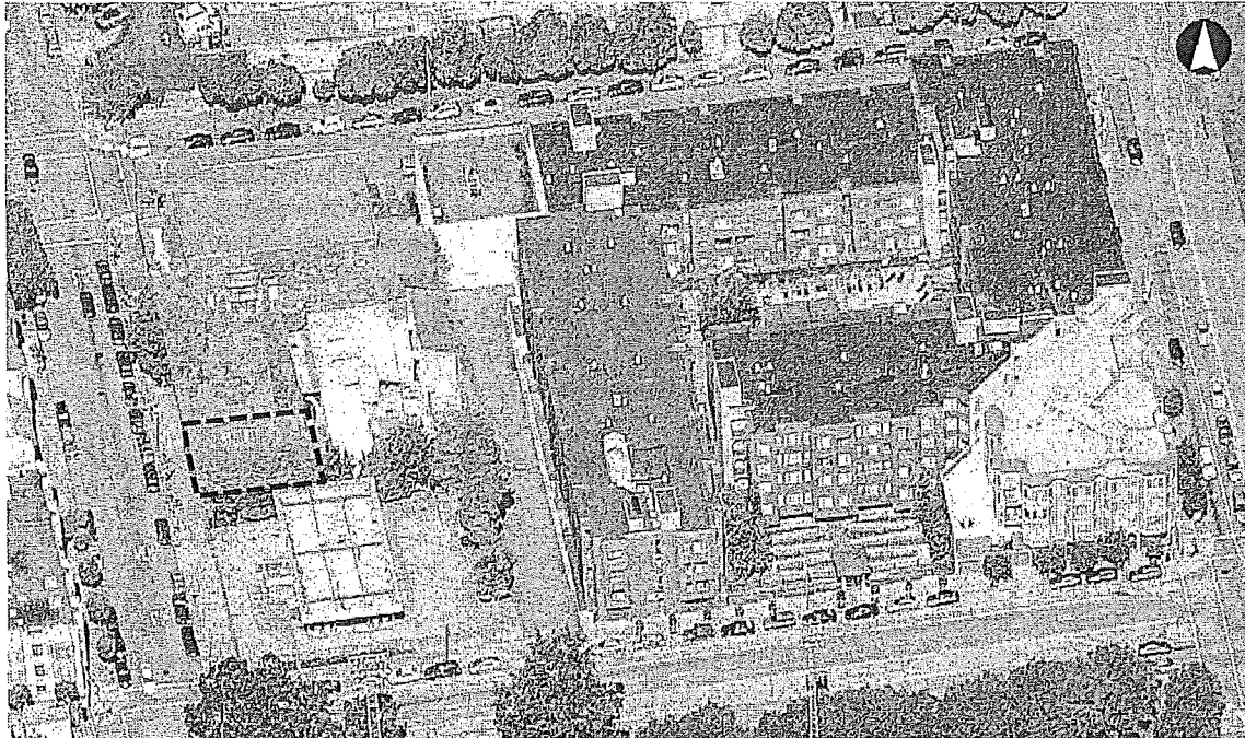
Figure 2: 3620 Buchanan Street, San Francisco, facing south. Yellow shading roughly delineates the subject parcel; black dashed outline roughly delineates the subject building.
