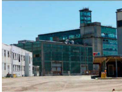
Northwest Elevation — Building 253
