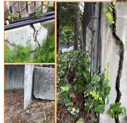
Cooling Tower foundation (above) structurally unstable.
