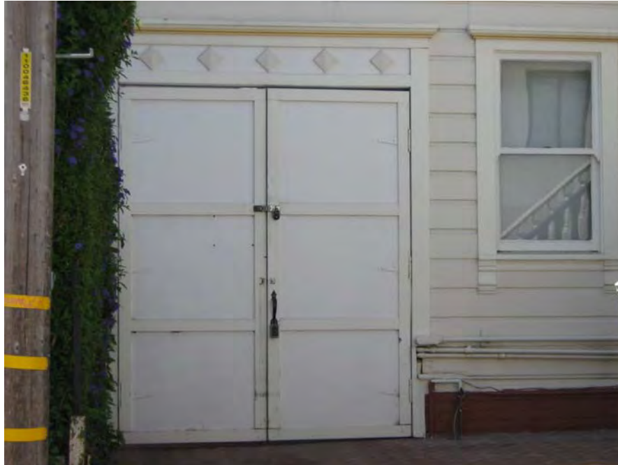
Left bay of the first floor at 156 Landers Street.
