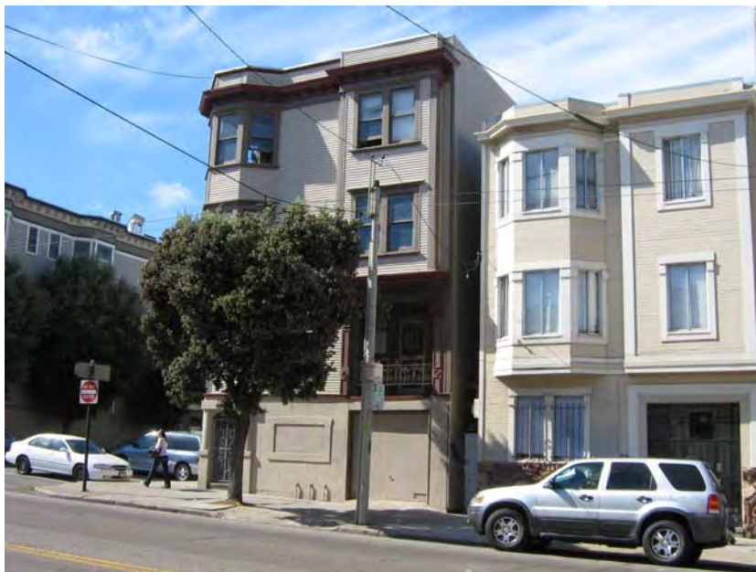
16 th Street (south) elevation
