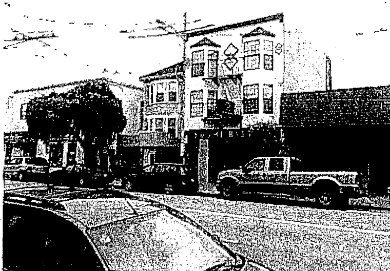
Subject property and buildings 100' to the East along Balboa Street
