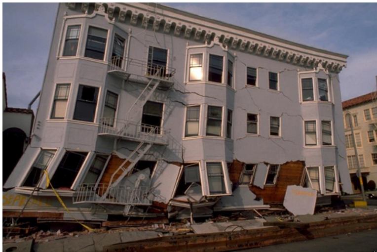
Damage from the 1989 Loma Prieta Earthquake
