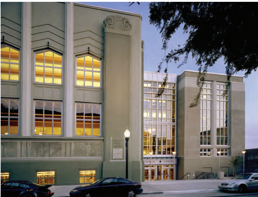
Figure 1. The addition to the right with its connecting hyphen is compatible with the Collegiate Gothic-style library. The addition is set back from the front of the library and uses the same materials and a simplified design that references, but does not copy, the historic building. Photo: David Wakely Photography.
