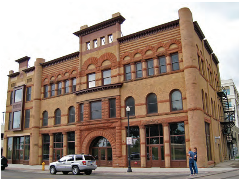
Figure 10. The small size and the use of matching materials ensures that the new addition on the left is compatible with the historic Romanesque Revival-style building.
