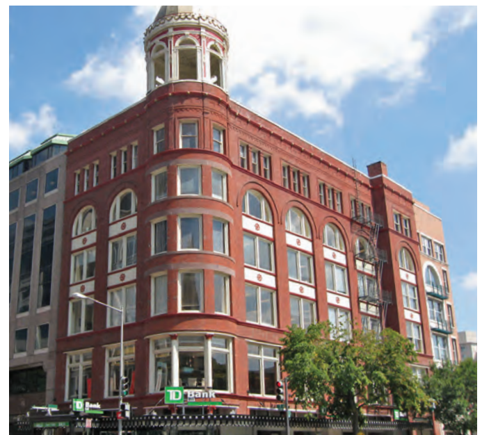
Figure 30. The small addition on the right of this late-19th century commercial structure is clearly secondary and compatible in size, materials and design with the historic building.
