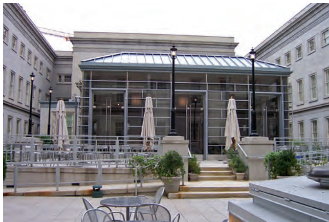
Figure 13. A glass and metal structure was constructed in the courtyard as a restaurant when this 1839 building was converted to a hotel. Although such an addition might not be appropriate in a more public location, it is compatible here in the courtyard of this historic building.
