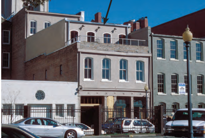
Figure 26. A rooftop addition would have negatively impacted the character of the primary facade (right) of this mid-19th century, four-story structure and the low-rise historic district. However, a third floor was successfully added on the two-story rear portion (below) of the same building with little impact to the building or the district because it blends in with the height of the adjacent building.
