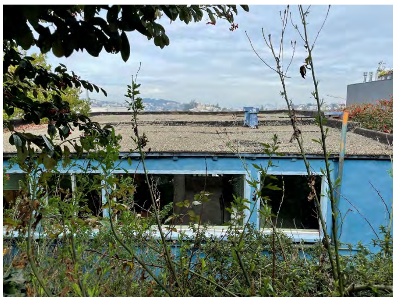
651 Duncan Street, rear elevation from rearyard, view north, 2020 Source: YA Studio
