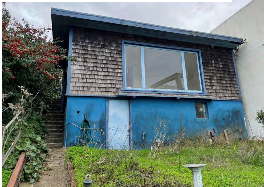
651 Duncan Street, front façade, view south, 2020 Source: YA Studio
