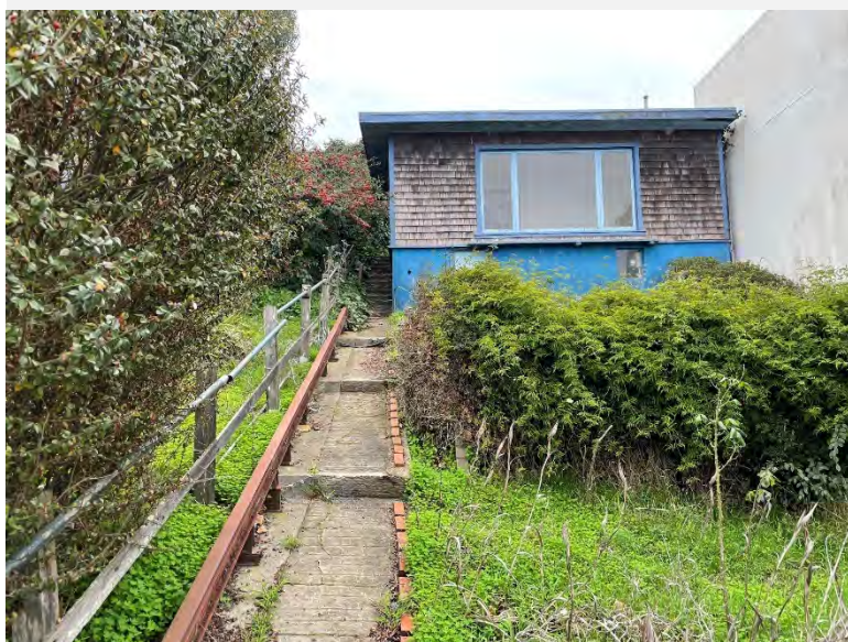
651 Duncan Street, front façade, view south, 2020 Source: YA Studio
