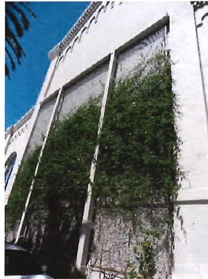
Figure 16. Structural metal frame with mesh screen and climbing vines on rear (south) façade. Source: Page & Turnbull, April 2019.
