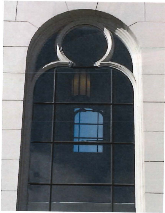
Figure 61. East façade, transept window after restoration. (Palisade Builders, 05/20/2018)
