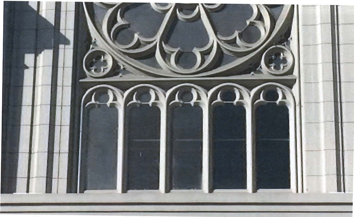
Figure 62. West transept rose window after restoration. (Palisade Builders, 05/20/2018)
