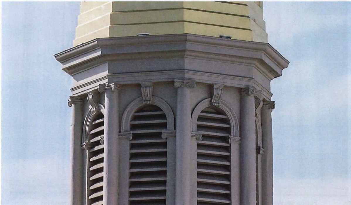
Figure 59. East tower detail after restoration (Rich Stapleton, 05/21/2018).
