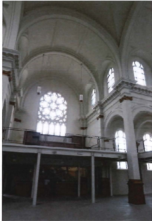
Figure 66. Interior view of west transept. (Page & Turnbull, 05/25/2018)
