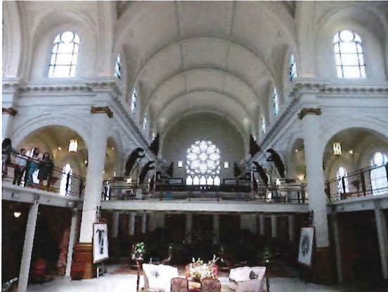
Figure 22. Non-original mezzanine along the aisles and spanning the nave, looking north. Source: Page & Turnbull, April 2019.
