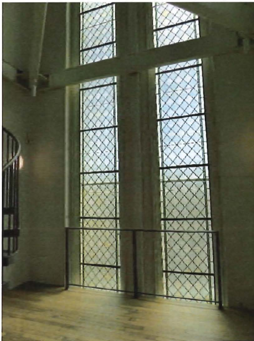
Figure 75. East tower, east windows after restoration (Page & Turnbull, 05/25/2018)
