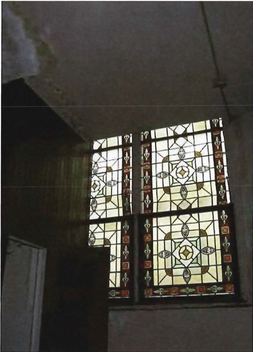
Figure 42d. Kitchen window, showing partition partially covering painted stained glass.
