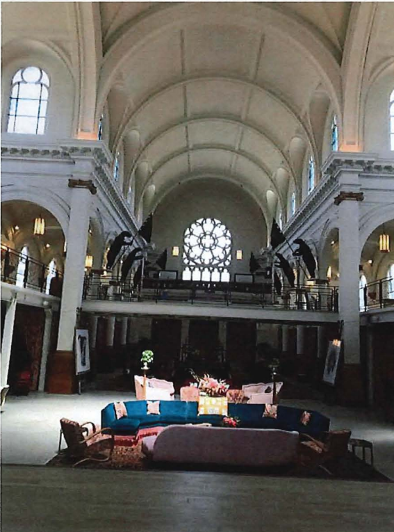
Primary interior volume facing northwest
