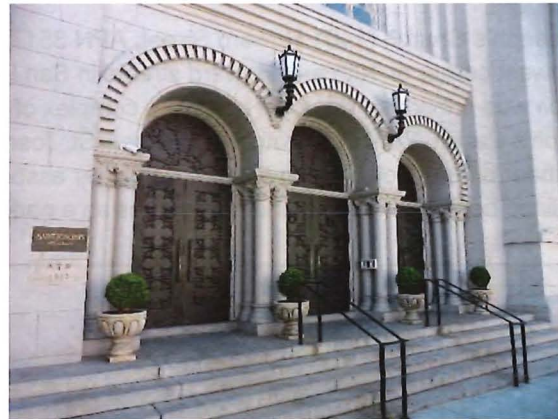
Figure 10. Main entrance to St. Joseph's Church. Source: Page & Turnbull, April 2019.
