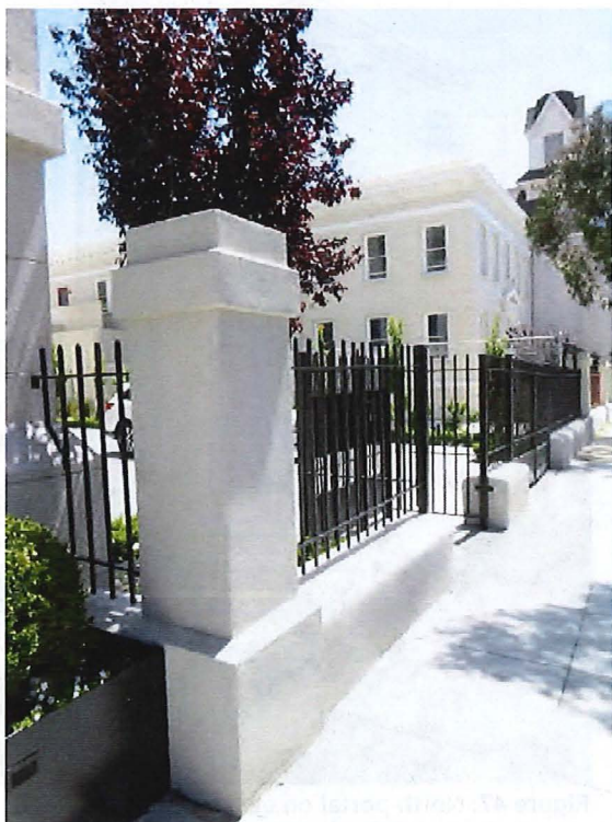
Figure 43. Perimeter fence and gate along Howard Street. View southwest. (Page & Turnbull, 05/25/2018)
