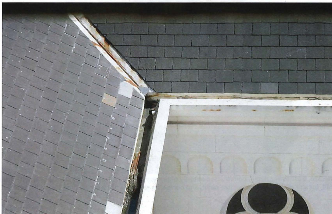
Figure 36c. Detail, corrosion and loss of paint and gilding at domes.
