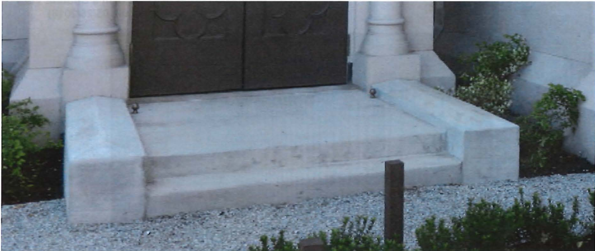
Figure 48. Detail, North portal stairs on east transept. (Page & Turnbull, 05/25/2018)
