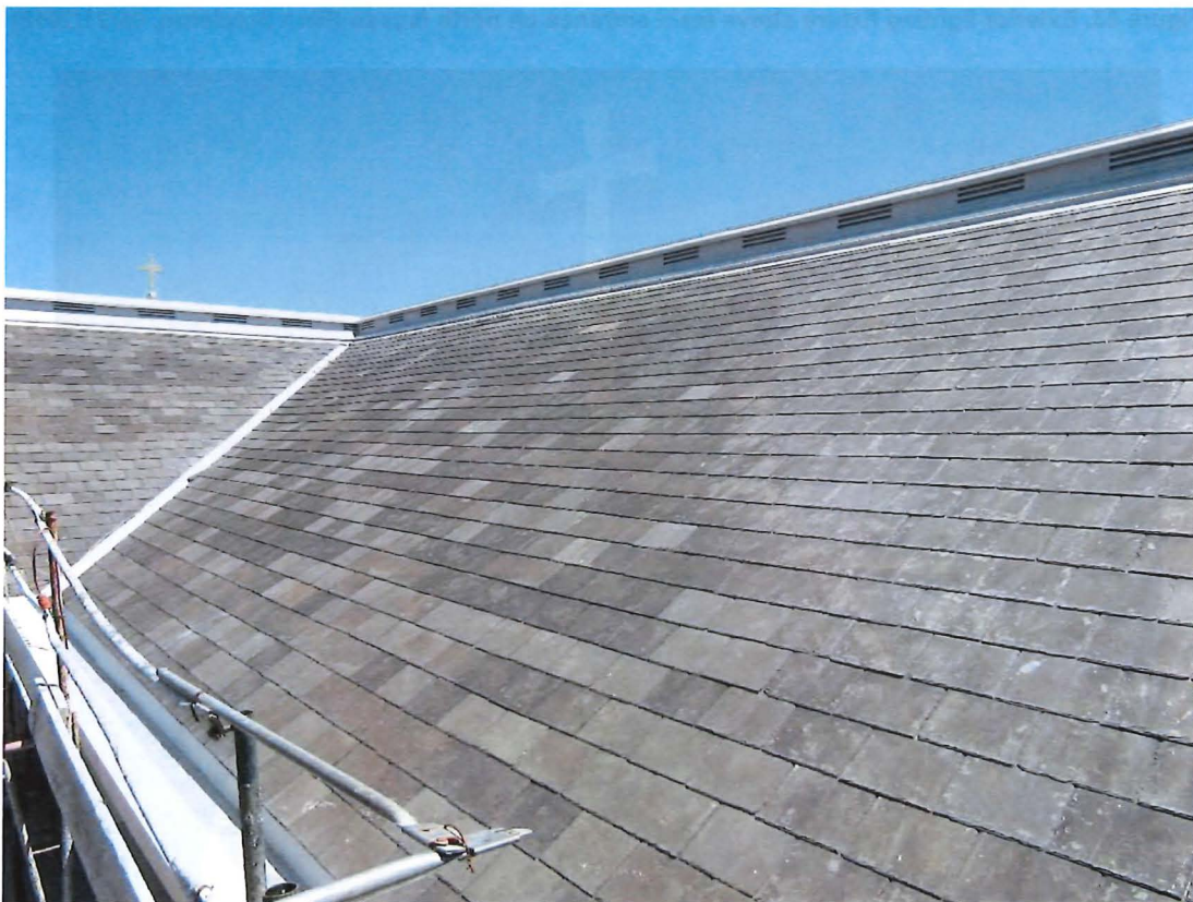
Figure 56. Main roof after restoration. (Palisade Builders, 05/20/2018)
