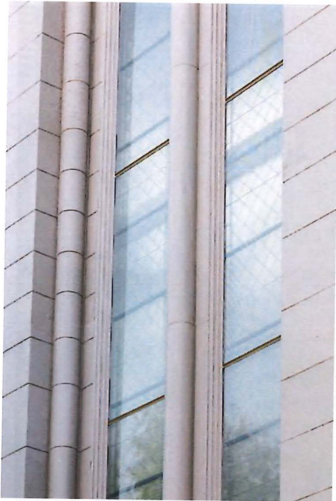
Figure 60. West tower, north window after restoration (Rich Stapleton, 05/21/2018).
