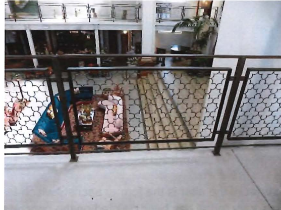
Figure 23. Mezzanine balustrade, looking down toward the nave. Source: Page & Turnbull, April 2019.
