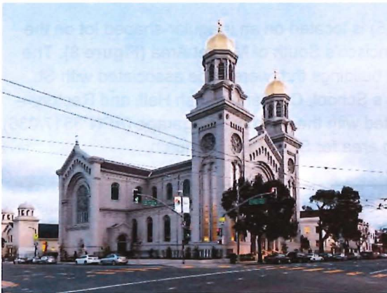
Figure 9. St. Joseph's Church. View south from Howard Street. Source: Rick Stapleton, September 2018.
