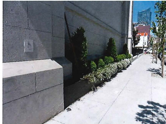
Figure 12. Contemporary steel planter at transept of east façade. Source: Page & Turnbull, April 2019.
