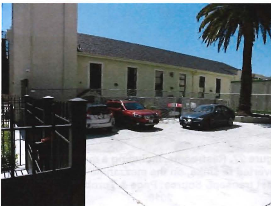
Figure 30. Concrete parking area southeast of St. Joseph's Church, at the former location of the garage, looking south.
