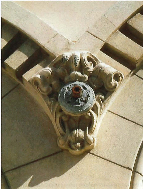
Figure 35b. Detail, original mounting hardware is all that remains in place.
