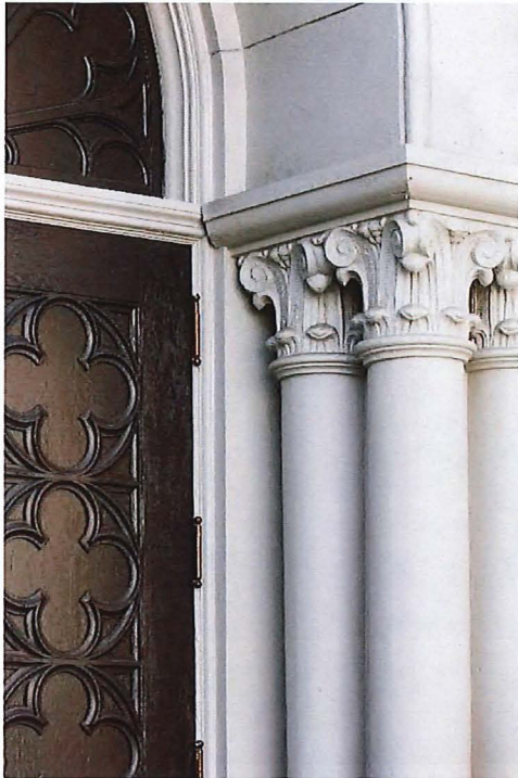
Figure 57. Column capitals at the main entry façade after restoration. (Rich Stapleton, 05/21/2018)
