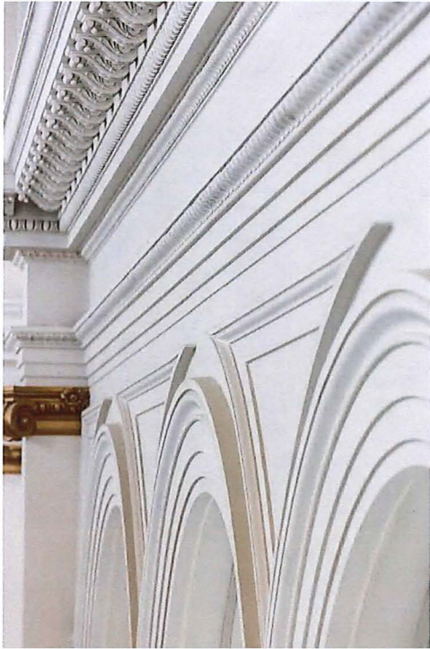
Figure 69. Detail, plaster arches. (Rich Stapleton, 05/21/2018)
