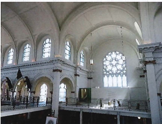
Figure 26. View of mezzanine level east transept. Restrooms are located behind the partial-height wall. Source: Page & Turnbull, April 2019.
