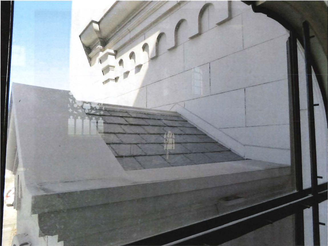
Figure 51. East façade, showing stucco condition after restoration (Page & Turnbull, 05/25/2018)
