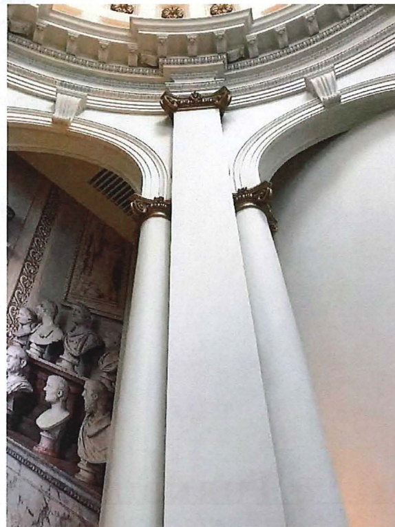
Detail of restored decorative plaster elements
