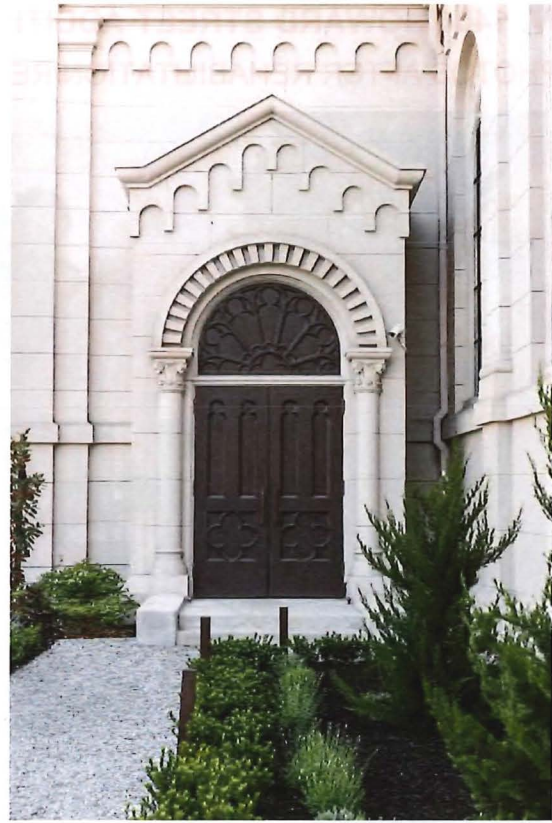
Figure 47. North portal on east transept. (Page & Turnbull, 05/25/2018)
