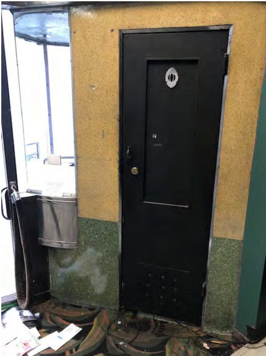
Clay Theater, ticket booth, view from lobby, 2022 Source: San Francisco Planning Department
