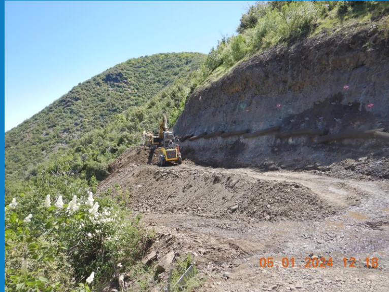
Adit 8/9 Cut Wall
