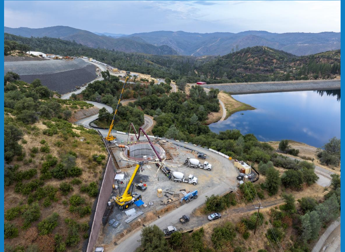
Flow Control Facility Location
