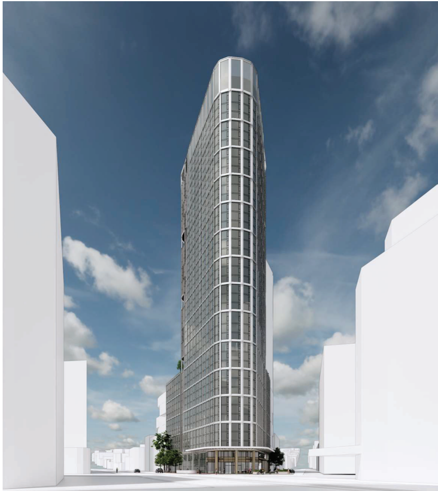
VIEW FROM MARKET LOOKING WEST
