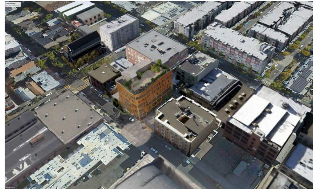
AERIAL VIEW FROM NORTH EAST - WITH NEW BUILDING
