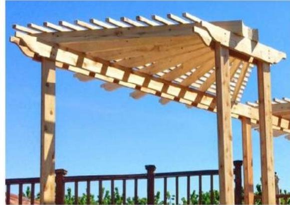
Exposed Cedar for Trellises at Courtyard and Roof Sealed, Clear
