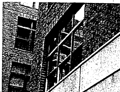
An good example of the use of brick with simply detailed windows relying on an ample recess as the major window detailing feature.
