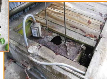
Cooling Tower failing structure (above) and rusted out sump (below)
