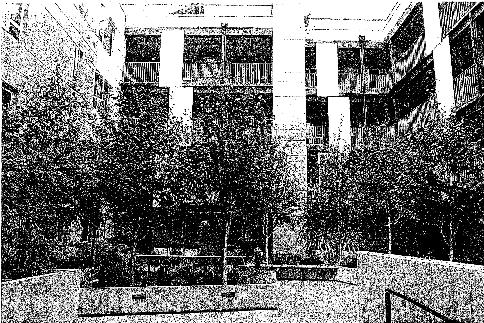
Bioretention planters are a central fixture in a courtyard area. Photo: Krystal Zamora
