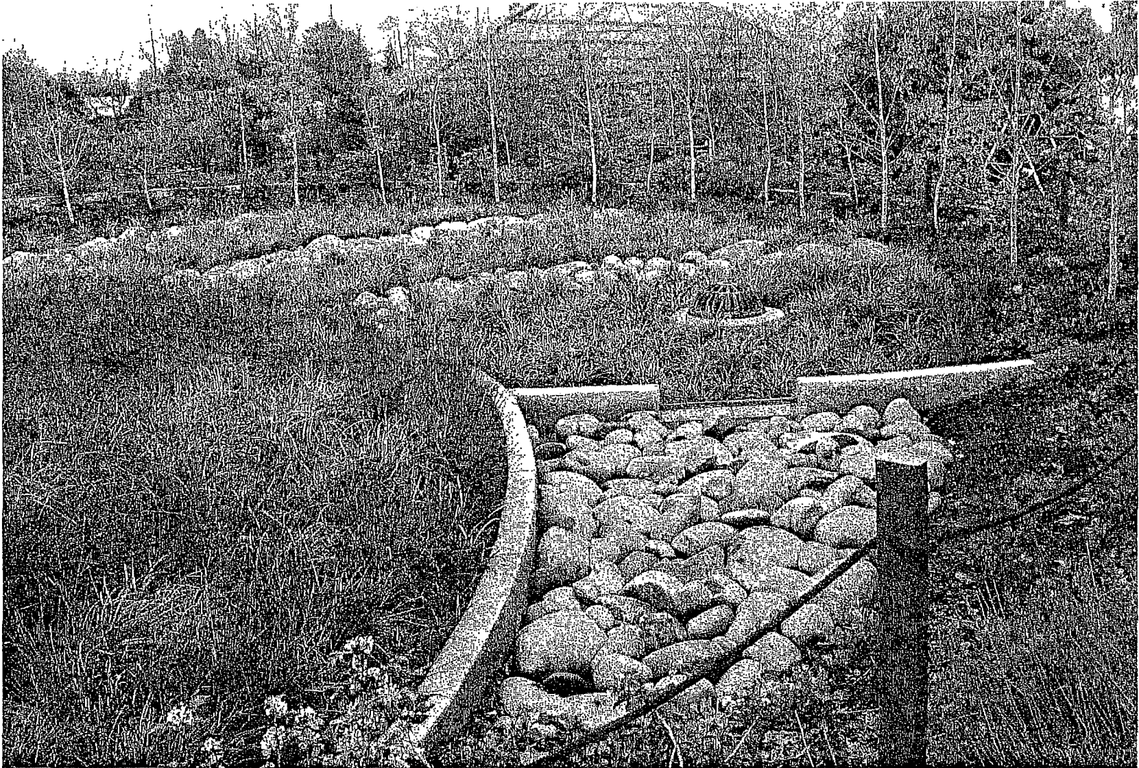
A rain garden at Glencoe Elementary in Portland, Oregon reduces stormwater flows to Portland's wastewater collection system. Photo: Rosey Jencks
