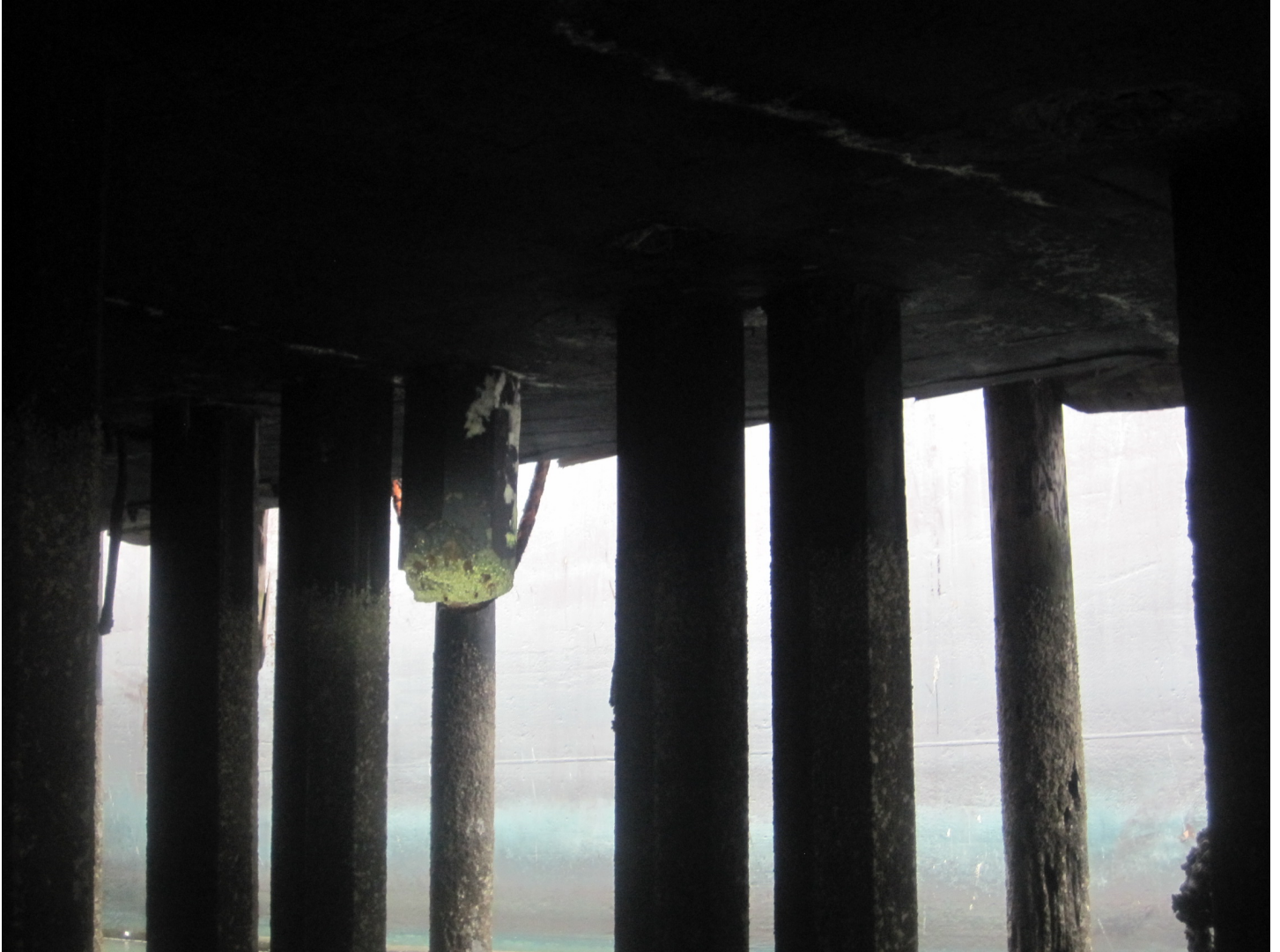
Photo 5. Missing pile
