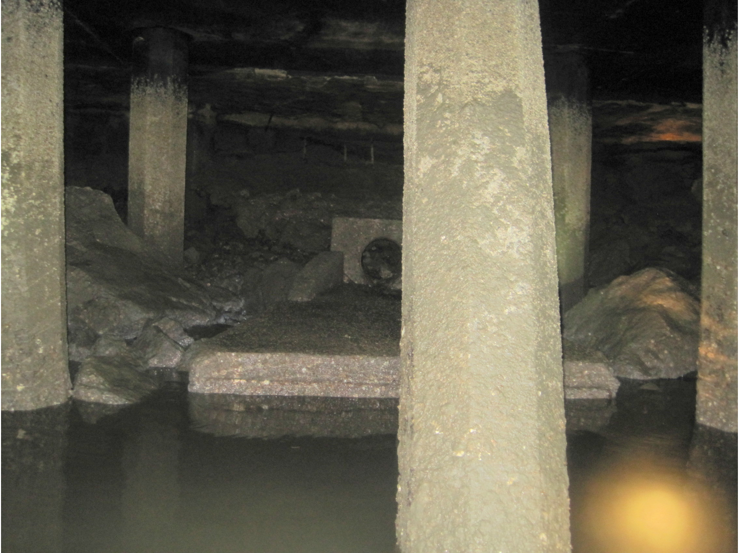
Photo 2. Drain underneath seawall
