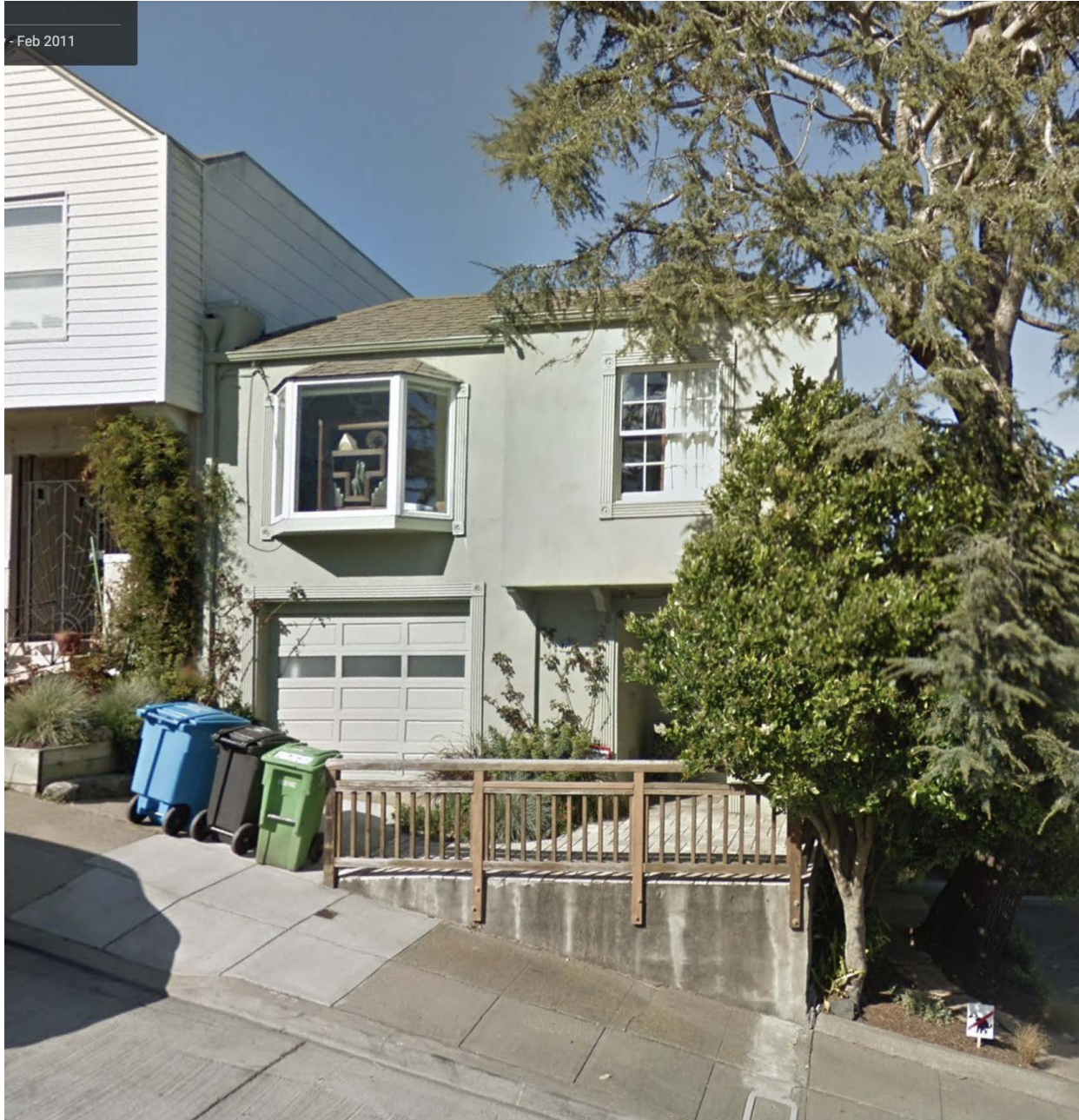
Photo#1 Original House prior to 2012 sale and Alteration permit.
