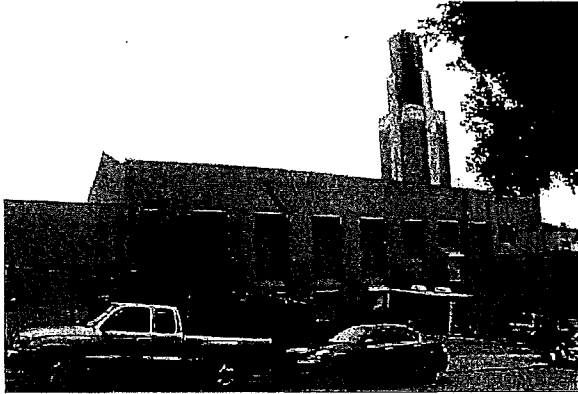
Figure 16. West wall of auditorium, looking southeast. Source: Christopher VerPlanck
