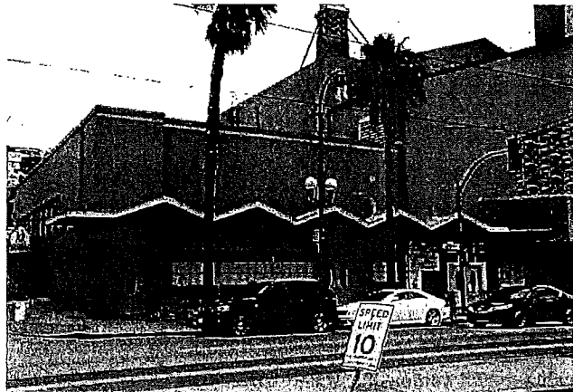
Figure 7. South wall of west retail wing, looking north. Source: Christopher VerPlanck
