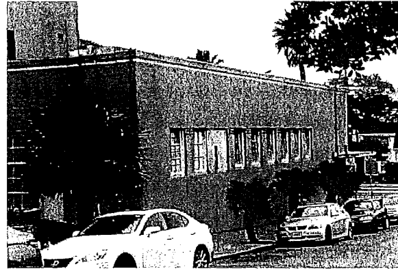
Figure 17. West wall of west retail wing, looking south. Source: Christopher VerPlanck
