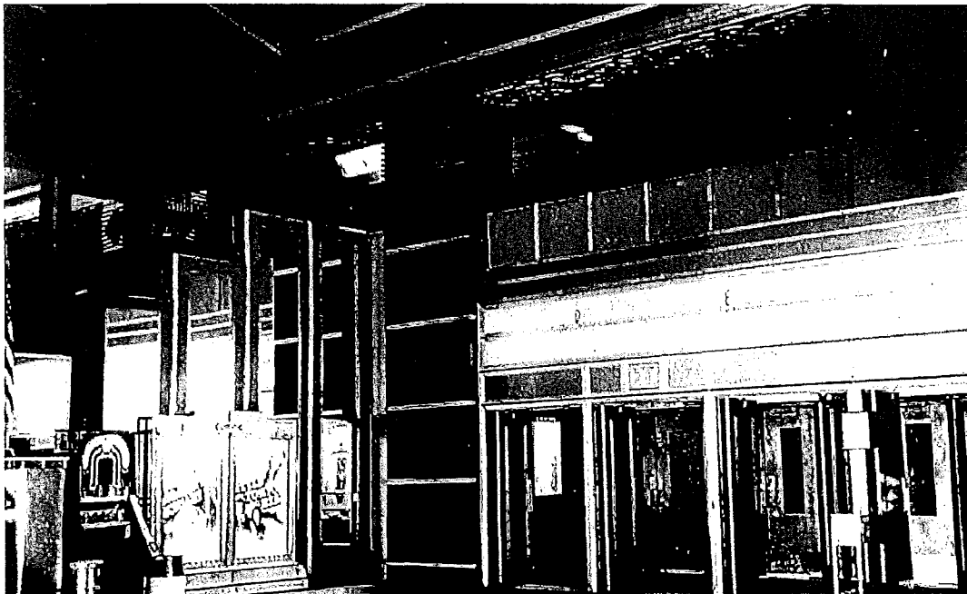
Figure 30. El Rey Theater Lobby, looking southeast, 1942.
