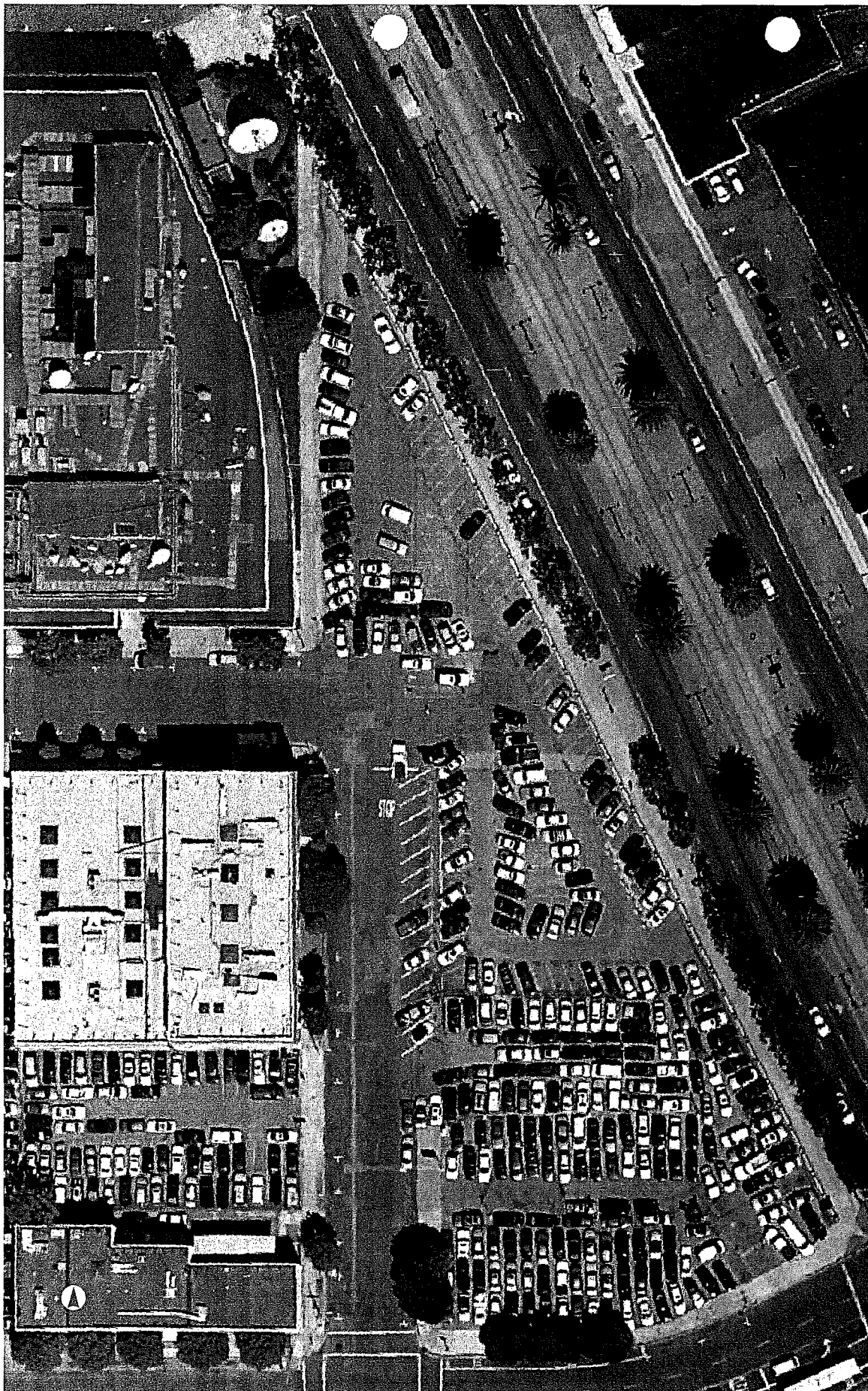
FIGURE 13 AERIAL VIEW OF THE EMBARCADERO: BROADWAY TO JUST SOUTH OF GREEN STREET
