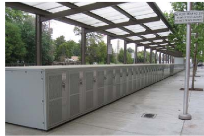
Example of Caltrain storage units
