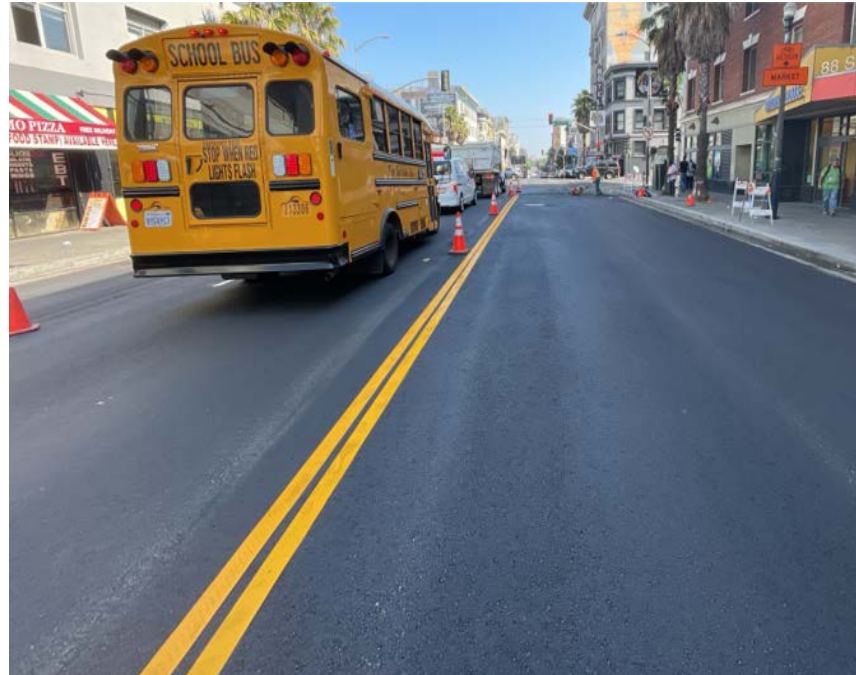
6th and Mission: New asphalt paving
