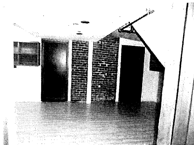
Basement with drop ceiling
