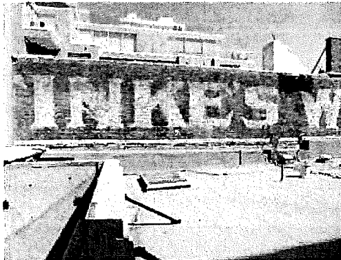
Roof, looking north
