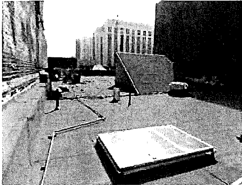
Roof overall, looking east
