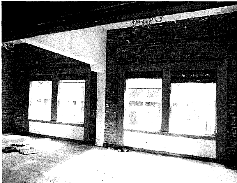
Interior of 2 nd Floor Montgomery Street windows
