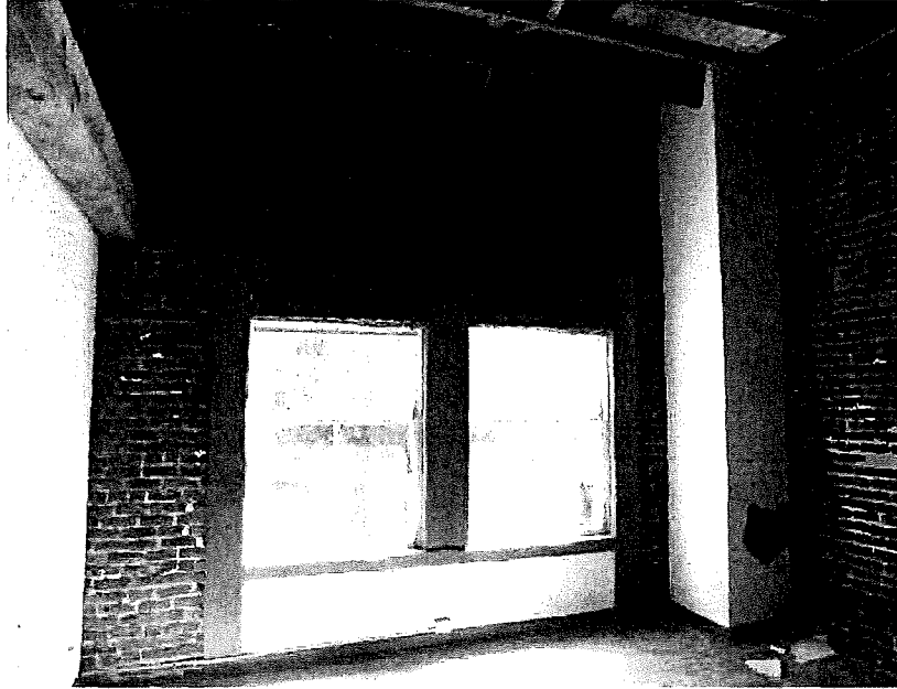
Interior of Montgomery Street 2 nd Floor windows
