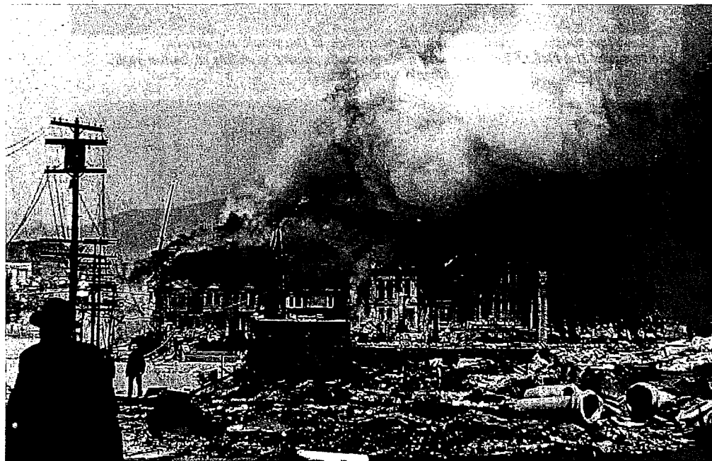
Fire at the corner of Van Ness Avenue and Vallejo Street. (Bancroft Library)
