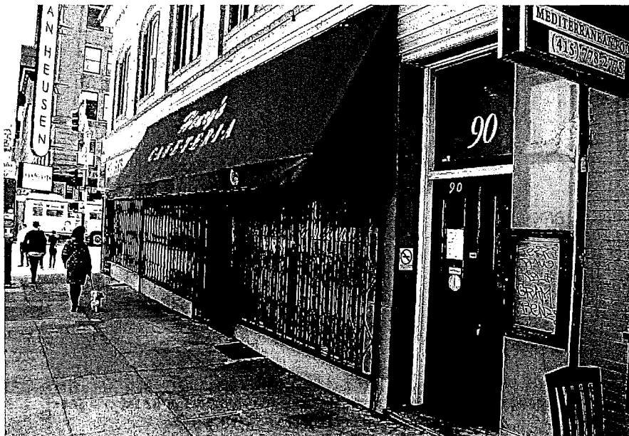
View toward Mission Street along the Second Street facade.
