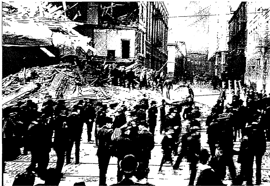
Rescue efforts at the Wilcox House, located only 75 feet north of the Bourdette Building at the southwest corner of Second and Jessie streets. The large building on the left beyond the wreckage is the Crossley Building. At right in the distance are the rear facades of the Grand Hotel and Palace Hotel. (Bancroft Library)
