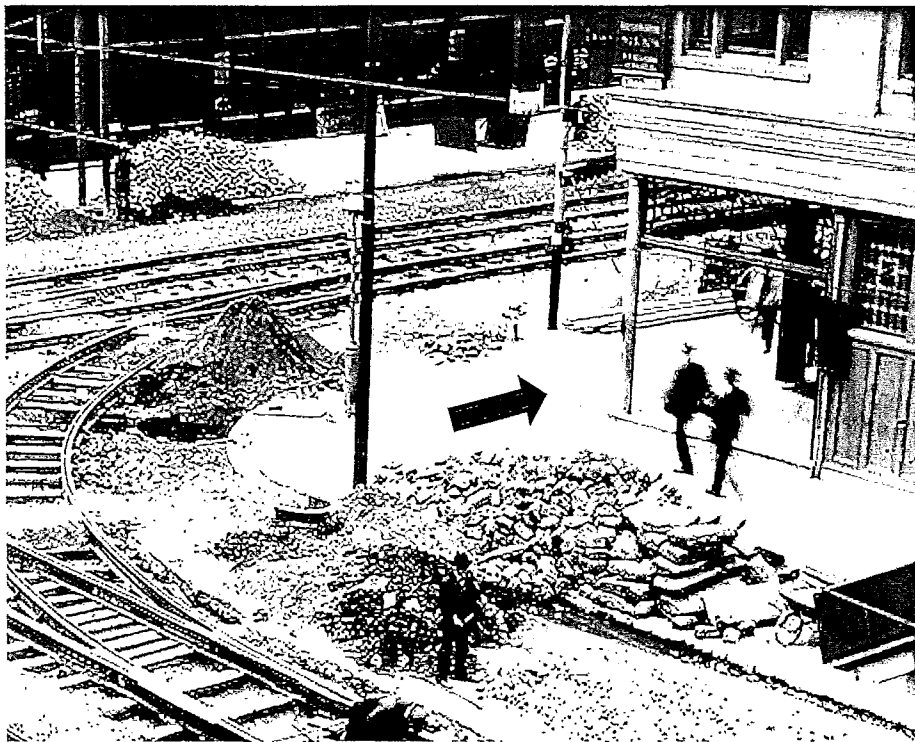
View of track construction at the intersection of Mission at Second Street, July 27, 1904. The Bourdette Building is at extreme right. Note the primary entry is open to the corner. (SFMTA Photo Archive)
