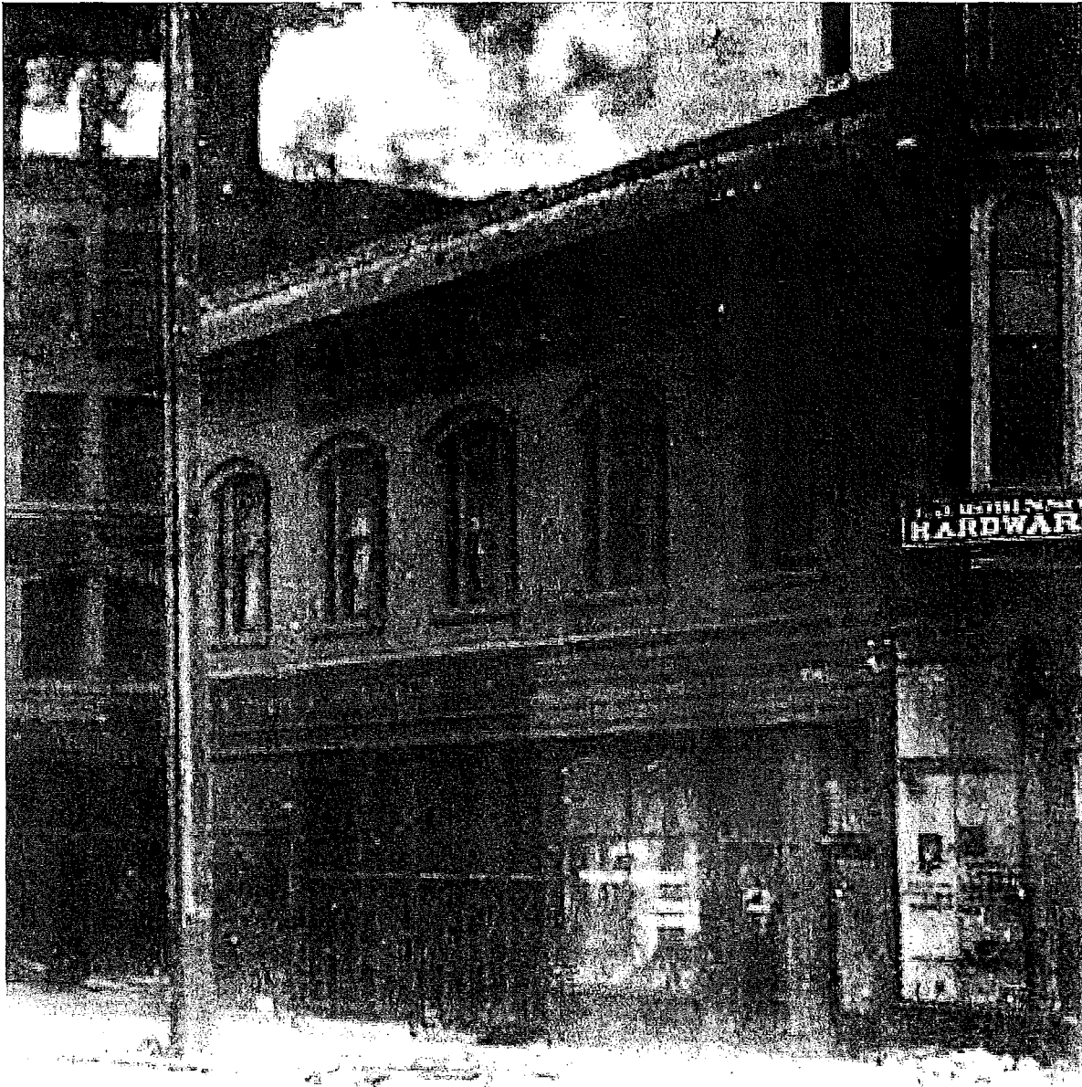
Detail view from the image on the previous page. This is the best photo available showing the original configuration of the Second Street storefront systems.
