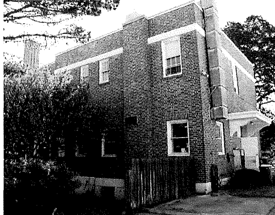
North elevation of service wing, April 2015
