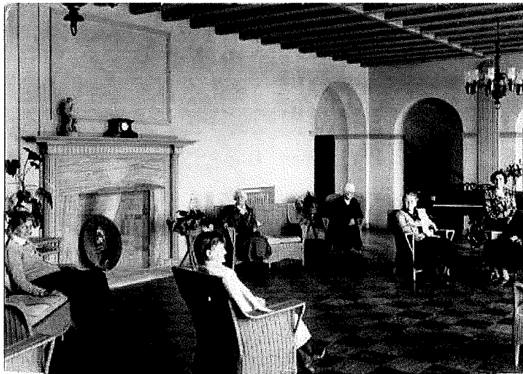
Living room of University Mound Old Ladies' Home shortly after construction (San Francisco Public Library, June 16, 1932)
