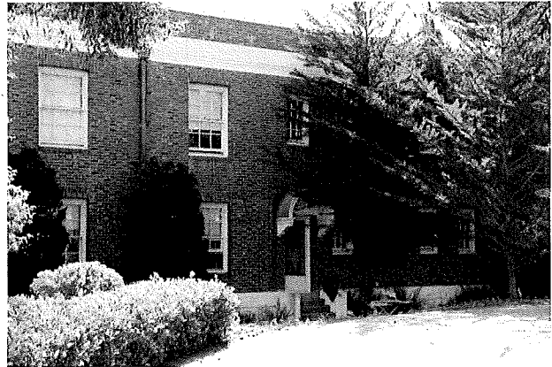
West elevation of south wing, April 2015
