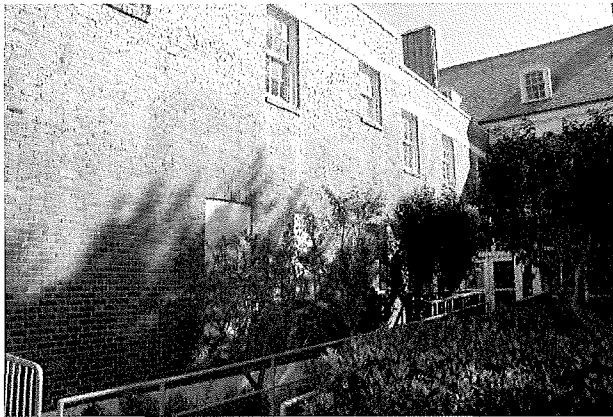
South elevation of service wing, April 2015
