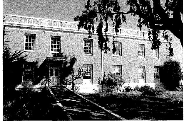
South elevation of south wing, April 2015
