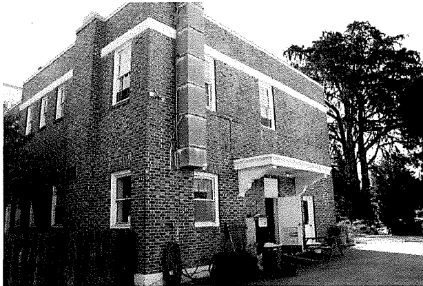
West elevation of service wing at right, April 2015
