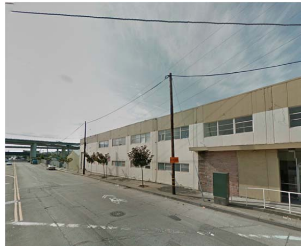
Figure 3. Photographs of Current Uses
