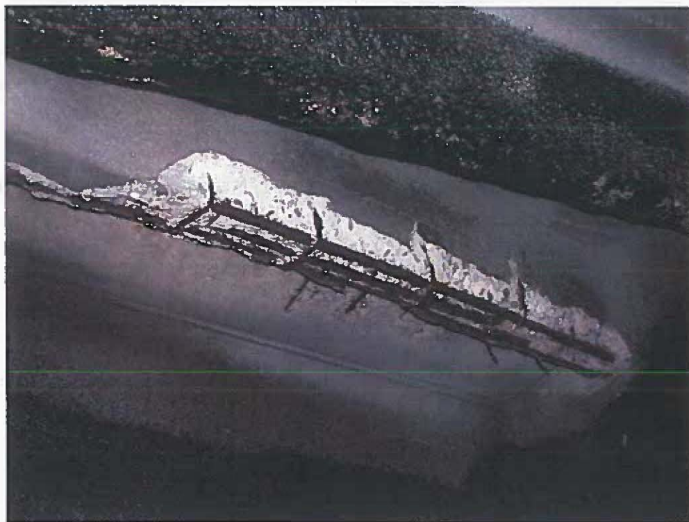
Figure 1 - Picture of Unrepaired Concrete Beam (Taken 5/14/19)
